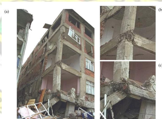
Fig. 1.1. Partial Building Collapse due to failure of beam-column joints in the Izmit, Turkey earthquake of August 17, 1999, (b) close-up of third-level joint, (c) close-up of second-level joint, (Courtesy of NISEE, University of California, Berkeley)
