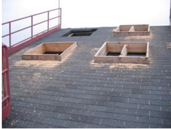
Figure 2.9: Roof ventilation panels (Source: Berks County Fire Training Centre, 2008)
