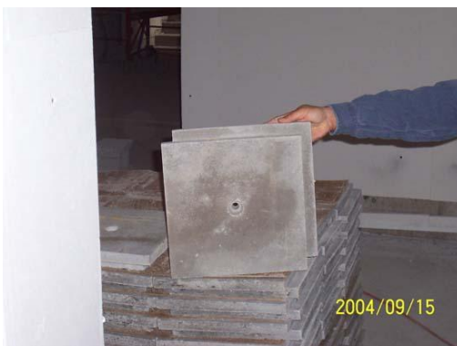
Figure 2.21: Concrete slabs used for the walls and ceilings of the burn building (Source: Berks County Fire Training Centre, 2008)
