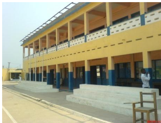
Figure 4.2: Front view of the main administration block
