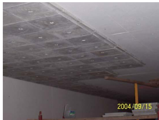
Figure 2.21: Concrete slabs used for the walls and ceilings of the burn building (Source: Berks County Fire Training Centre, 2008)
