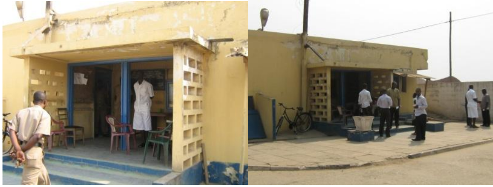
Figure 4.10: The sub fire station at the school
