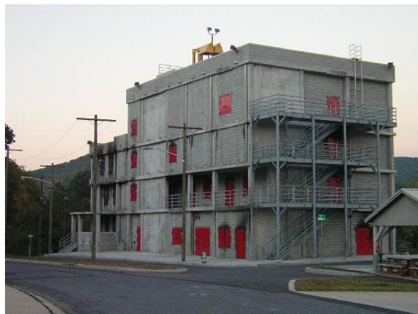
Figure 2.10: The live fire burn building (Source: Berks County Fire Training Centre, 2008)
