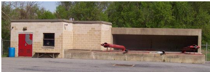
Figure 2.14: Drafting pit (Source: Berks County Fire Training Centre, 2008)
