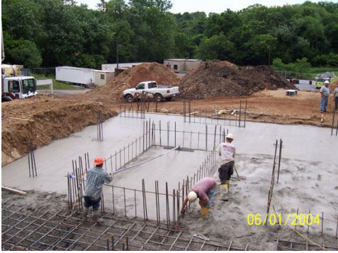
Figure 2.19: Casting of ground concrete floor slab (Source: Berks County Fire Training Centre, 2008)
