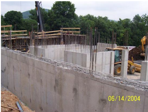
Figure 2.20: Erection of concrete walls reinforced with steel (Source: Berks County Fire Training Centre, 2008)
