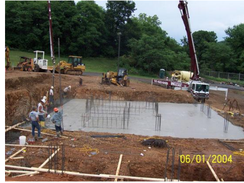
Figure 2.19: Casting of ground concrete floor slab (Source: Berks County Fire Training Centre, 2008)
