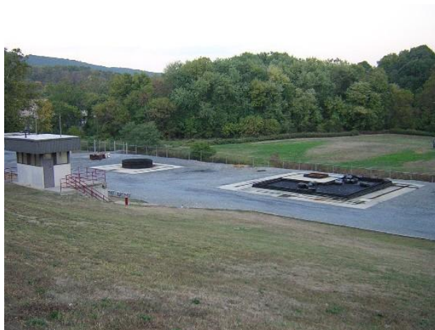
Figure 2.12: Flammable liquids pit (Source: Berks County Fire Training Centre, 2008)
