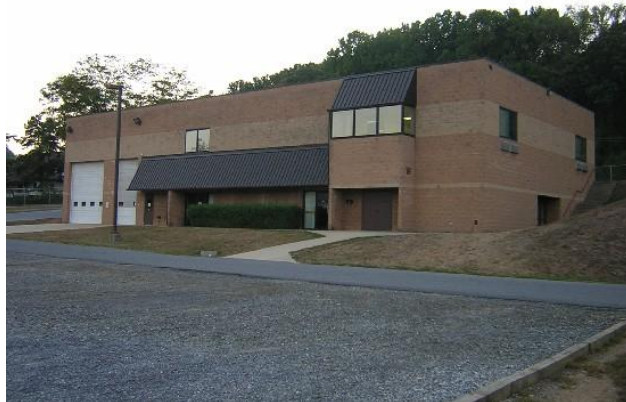
Figure 2.7: The administration building (Source: Berks County Fire Training Centre, 2008)
