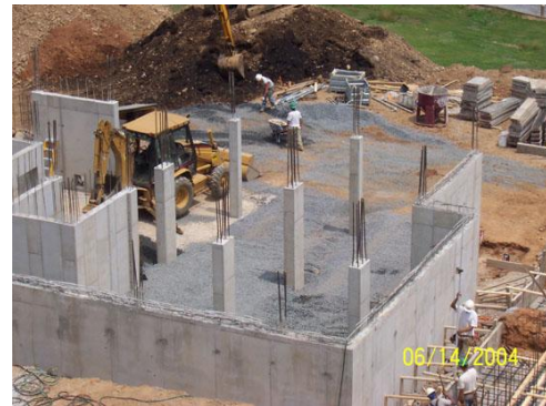
Figure 2.20: Erection of concrete walls reinforced with steel (Source: Berks County Fire Training Centre, 2008)
