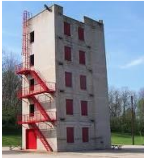
Figure 2.8: Drill tower (Source: Berks County Fire Training Centre, 2008)
