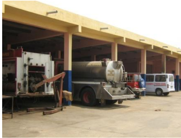
Figure 4.9: The maintenance department
