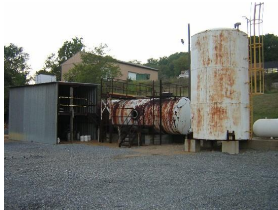
Figure 2.13: Confined space tank (Source: Berks County Fire Training Centre, 2008)
