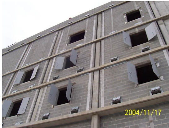
Figure 2.11: Burn building showing steel windows (Source: Berks County Fire Training Centre, 2008)
