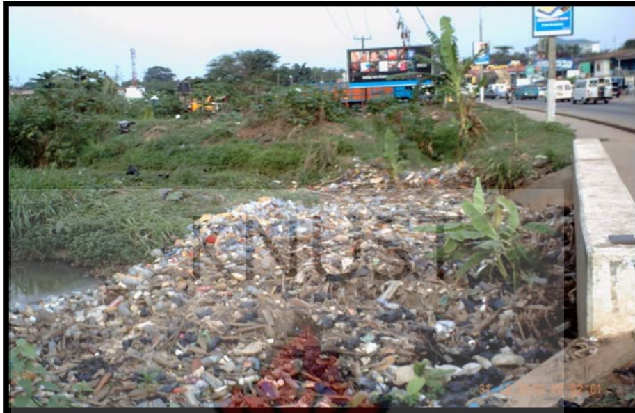
Figure 3.8: Picture showing choked culverts in the Aboabo river
