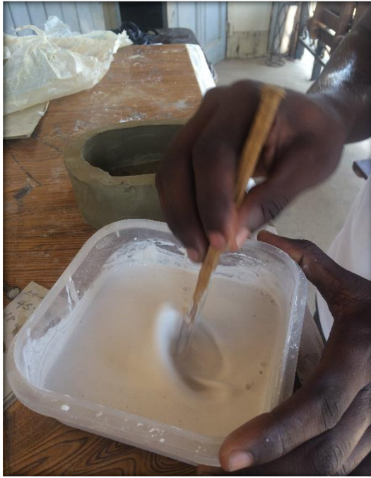
Plate 3.35: Shows the POP being stirred to become slurry
