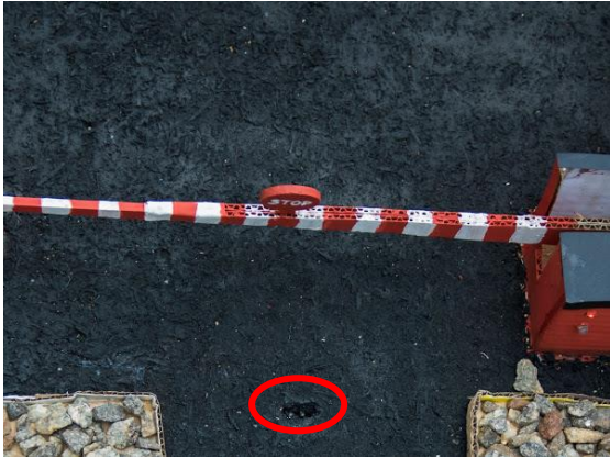
Plate 3.89: The circled component fixed in the road shows the infrared (IR) sensor
