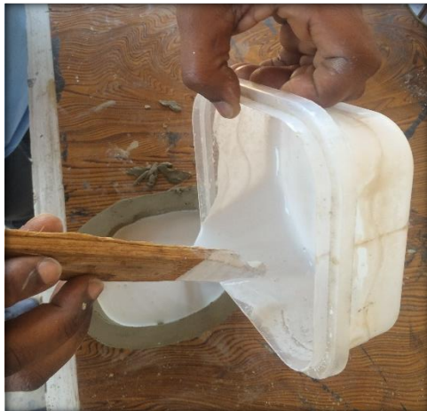
Plate 3.37: Shows the pouring of slurry POP into cavity.
