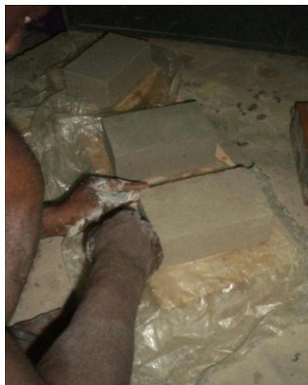
**Plate 3.52: Researcher dressing to fix little broken parts of the molded bricks**
