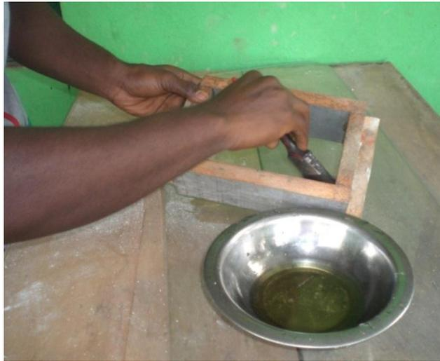
**Plate 3.48: Researcher lubricating the inner walls of the brick making mould with vegetable oil**
