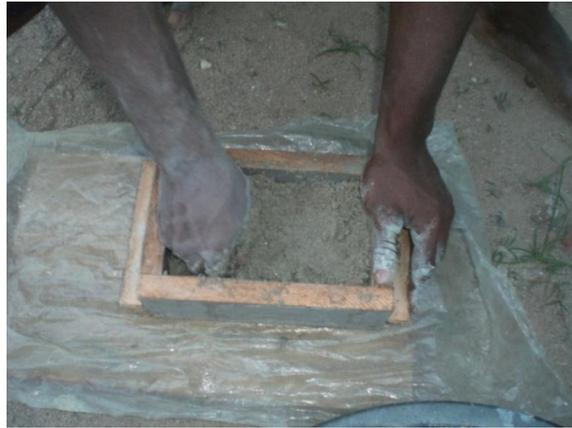
**Plate 3.50: Researcher pressing the composed body into the mould to make the brick**
