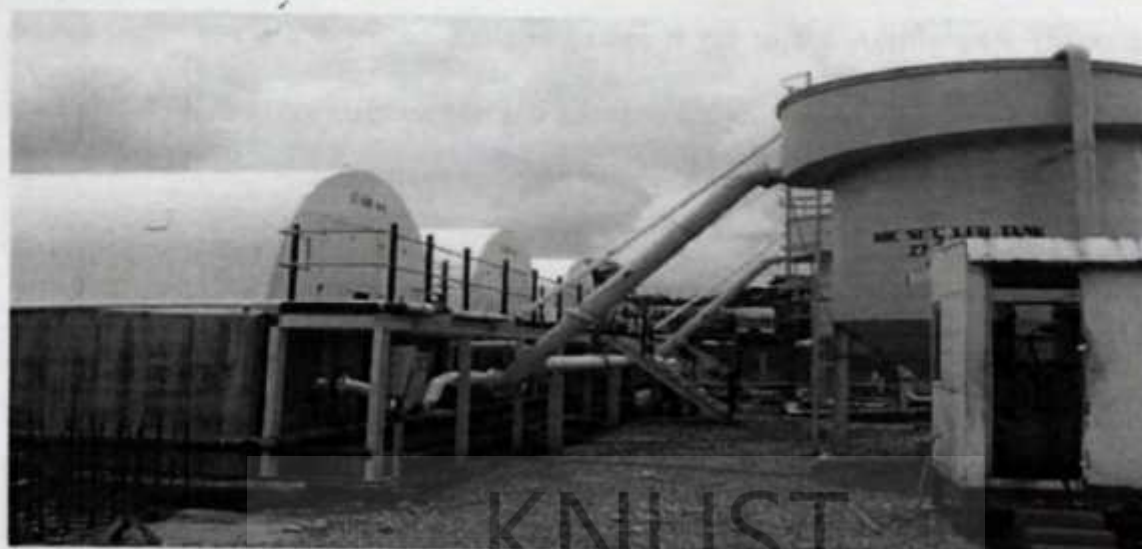
Figure 3-5: Settling tanks
