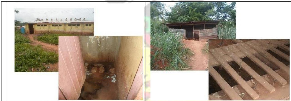
Plate 1: Latrines identified during assessment of sanitation facilities
