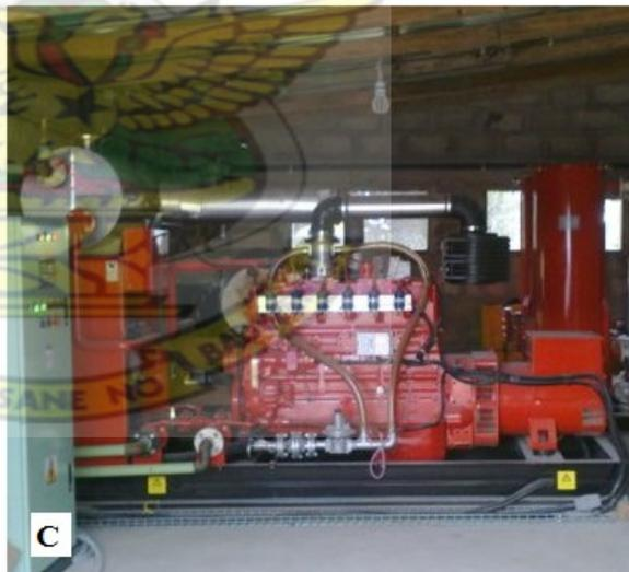
**Figure 3.10 Equipments that were ran on the biogas. A: Gas burner used for direct combustion of biogas. B: Boiler used for drying the fruits. C: Generator set**
