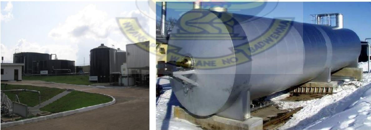
**Figure 2.5: High -TechAD Plants(Left) Vertical digester at Guinness Ghana Limited in Kumasi (Aklaku, 2011a) and (Right) Horizontal digester in Denmark (Al Seadiet *et al.*, 2008)**
