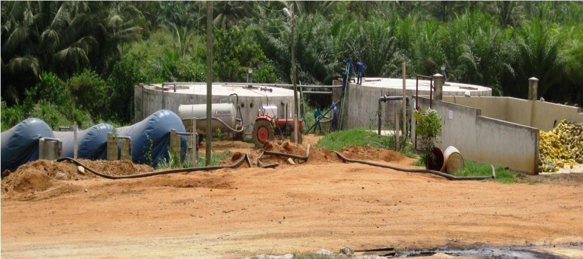
**Figure 3.4: The two 450 cubic meter (m<sup>3</sup>) AD plants constructed at the hpw Fresh and Dry Limited premises at Adeiso**
