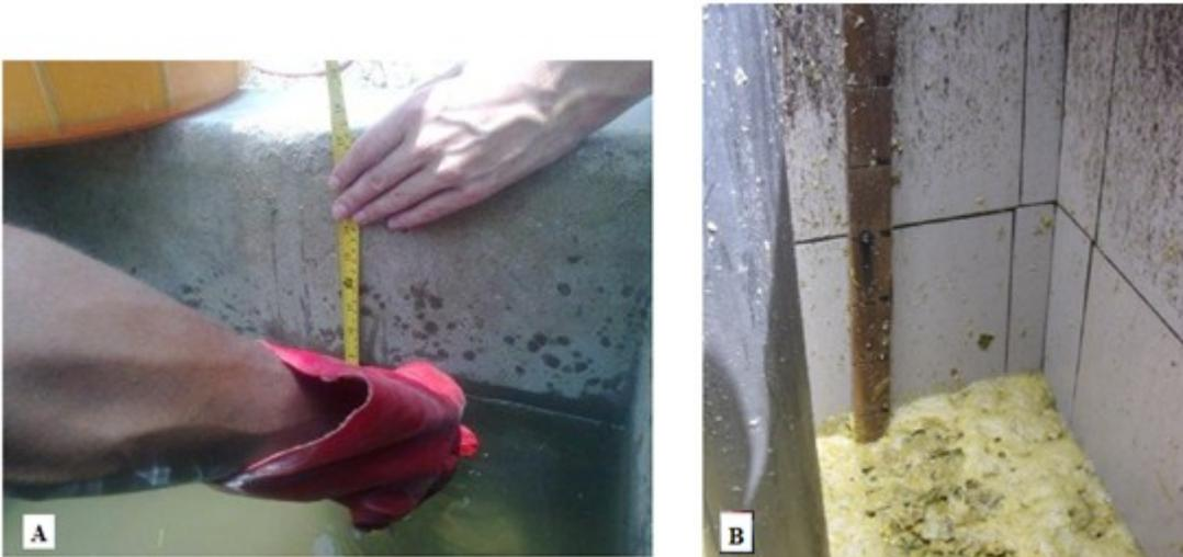
**Figure 3.6: Calibrated Mixing Chambers. A. One of the Site operators making a 25 litre mark on the mixing chamber wall at GIDA site. B. Wooden rule inserted in the mixing chamber at Adeiso (Picture by Johanna Grim & Maria Johansson)**
