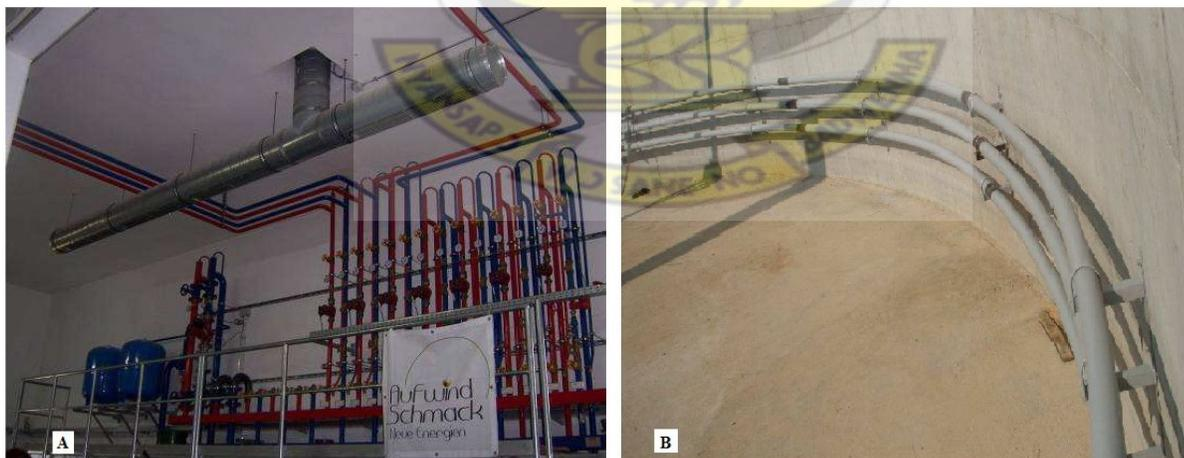
**Figure 2.7: The Heating System of a High-Tech Plant. A: The heating system of a high-tech digester and the heating pipes installed in the digester (Rutz, *et al.*, 2008 cited by Al Seadi *et al.*, 2008)**
