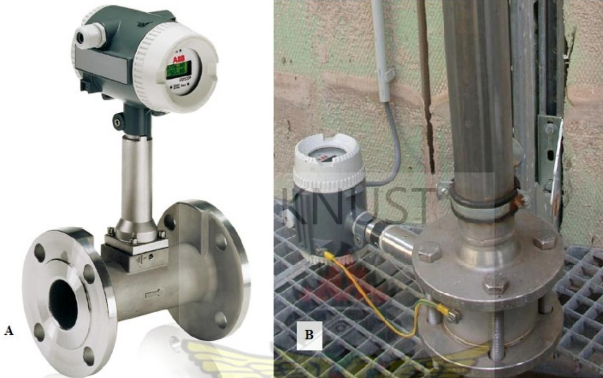
**Figure 2.20: Vortex Flow meter (left) Vortex flow meter connected to a digester(Adapted from ABB Vortex flowmeter)**
