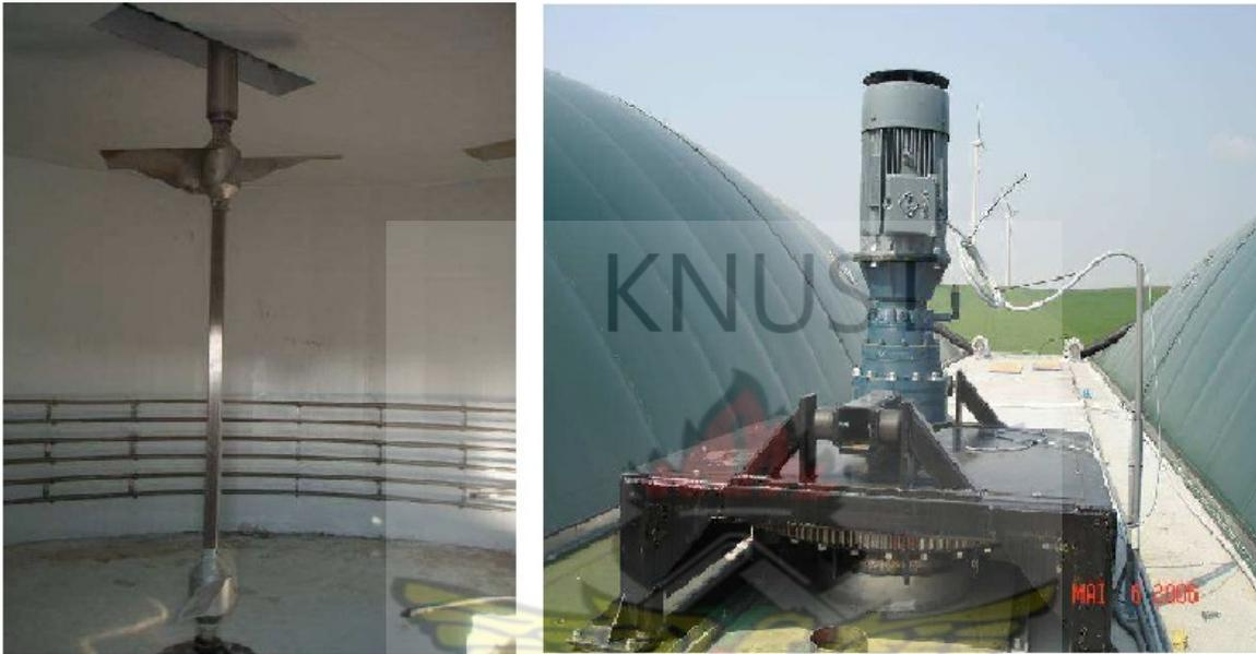
**Figure 2.6: Parts of the Mechanical Stirrer. (Left) Mechanical Stirrer and (Right) its stirring engine (Al Seadi *et al.*, 2008)**
