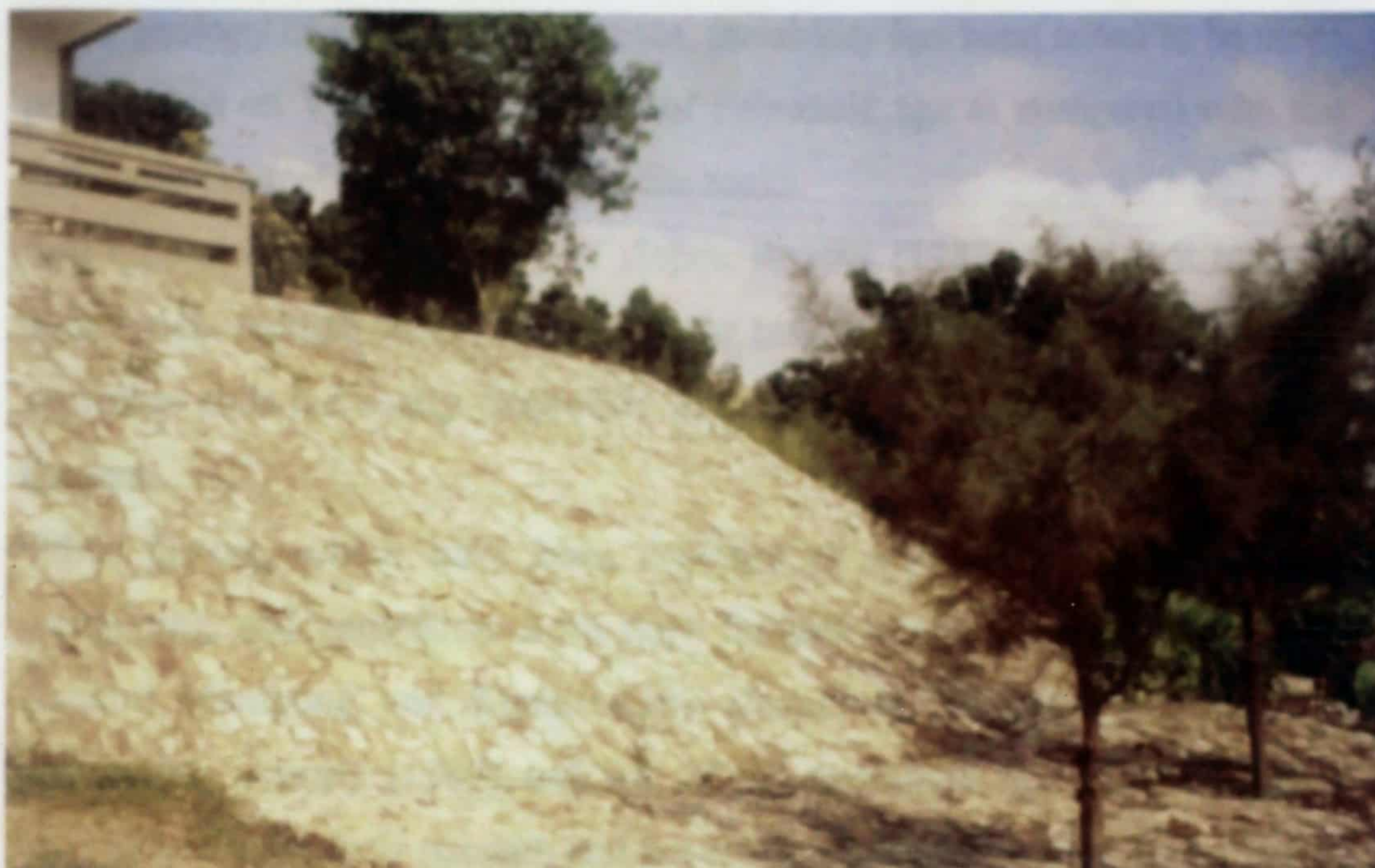
Photo 6: Unsympathetic Slope Stabilization in a Residential area
