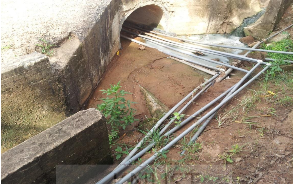
Plate 3: Series of distribution pipelines running through the main drains in Appiadu.
