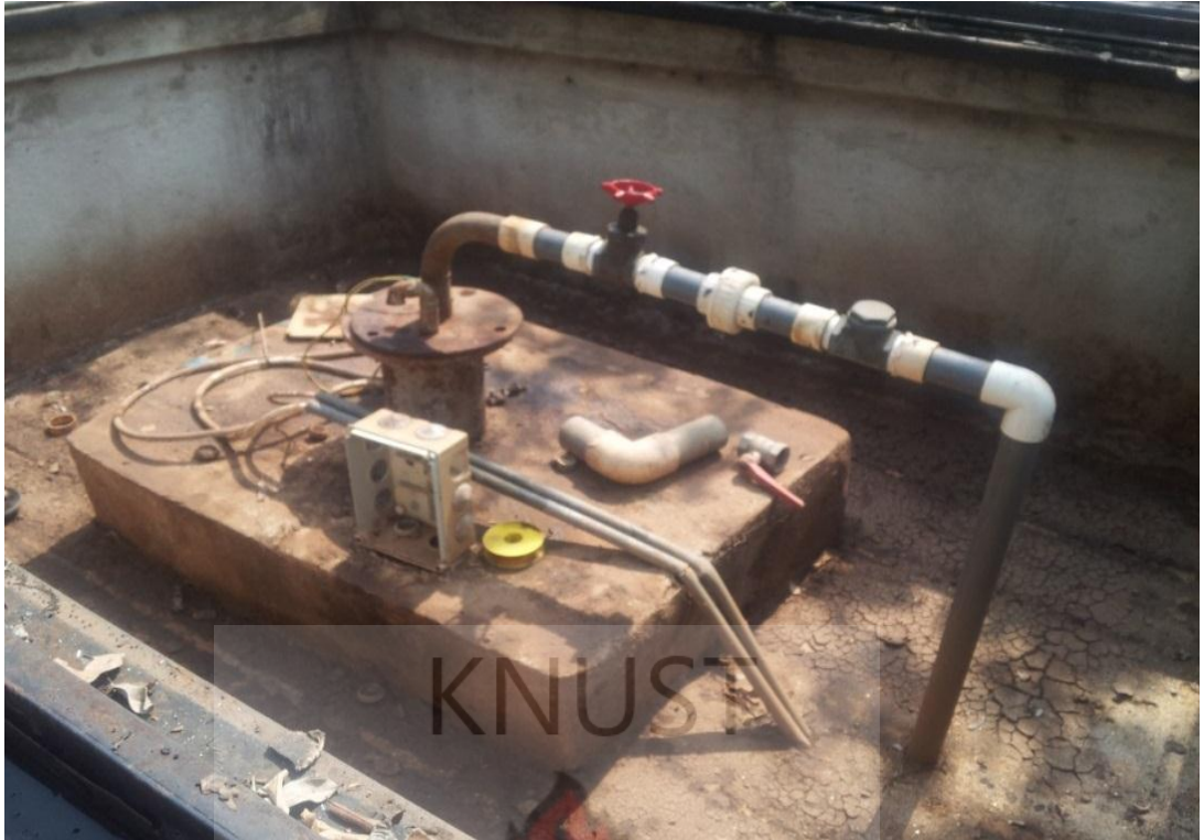
Plate 2: Borehole with pump used to draw groundwater in Appiadu
