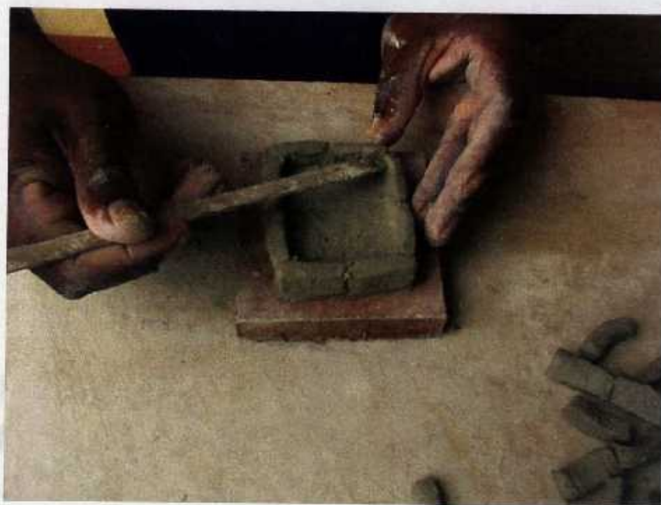
Plate 68 Raising walls by joining the bricks
