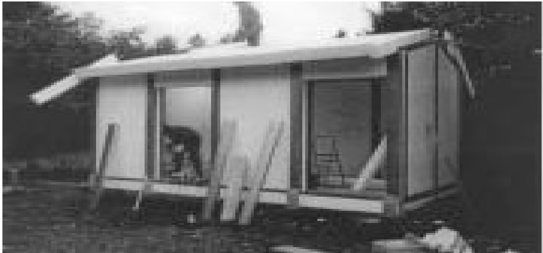
Plate 2.11: Metal Profiles and Expanded Polystyrene Core Wall system
