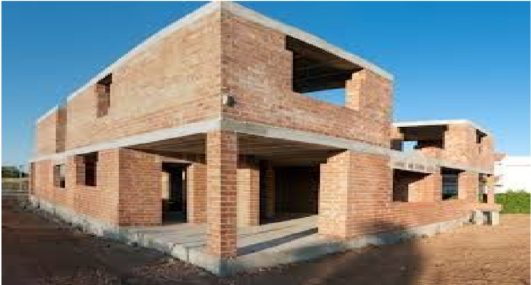
Plate 2.3: Massive Wall System with Burnt Bricks
