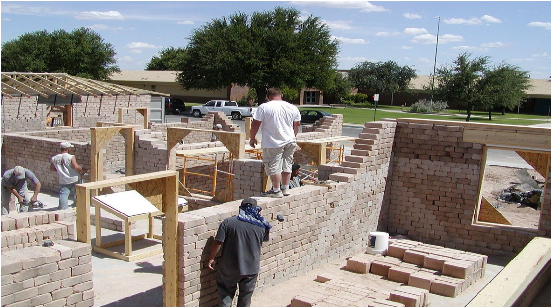
Plate 2.1: Massive Wall System with Compressed Earth Blocks
