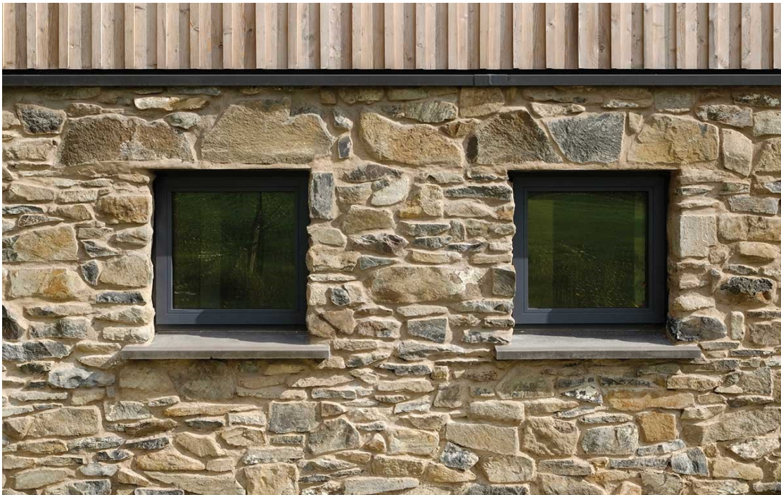
Plate 2.4: Massive Wall System with Stones
