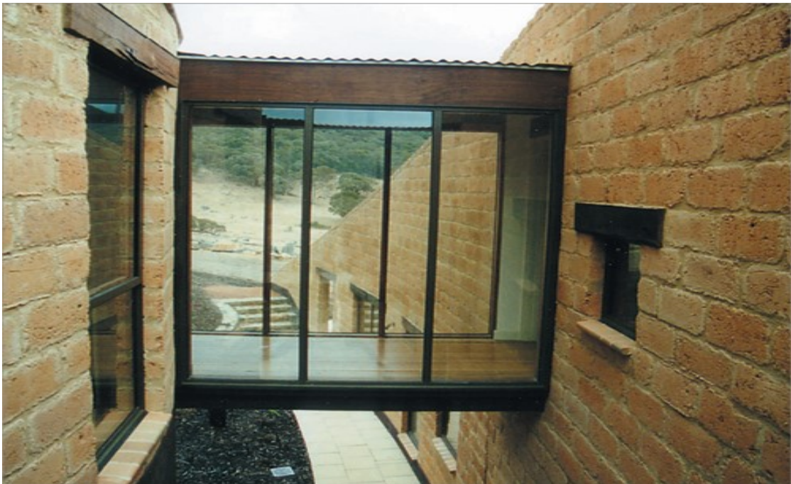
Plate 2.2: Massive Wall System with Mud Bricks
