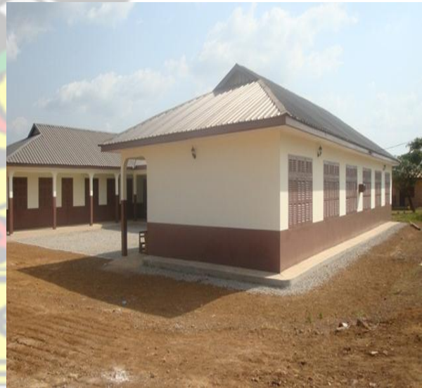
Figure 4.6 Six Classroom Block at Wamahinso
