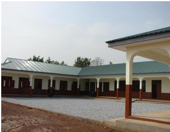
Figure 4.3 Six Classroom Blocks at Kenyasi No2
