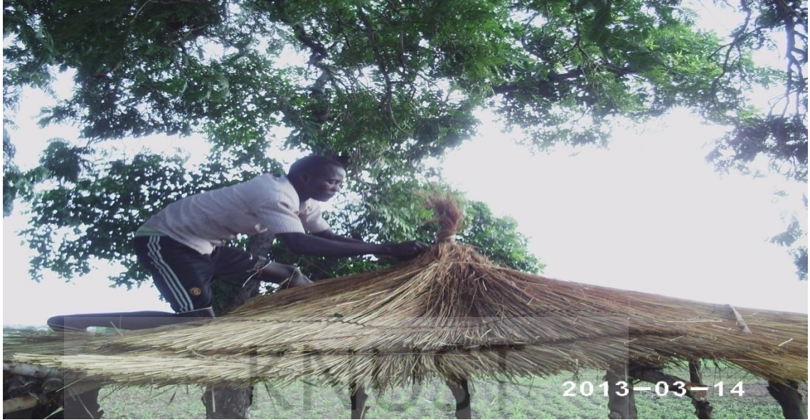
Plate 1: Roofing the evaporative cooler
