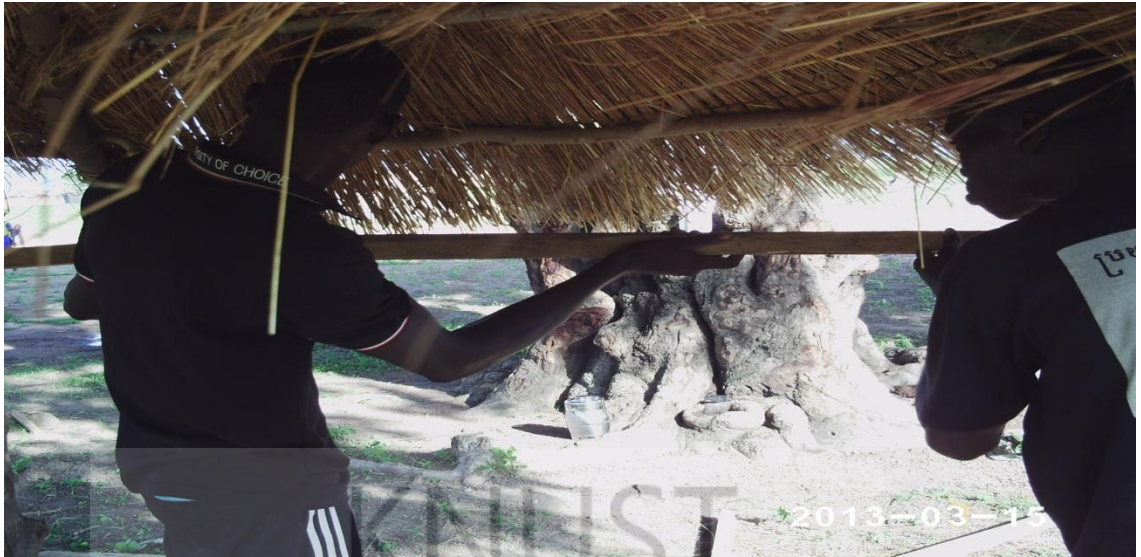
Plate 3: Constructing the structure
