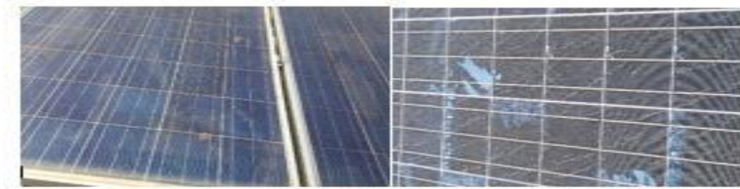
Plate 4- 4: front glass slightly soiled
