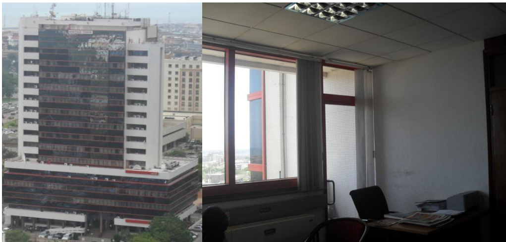
Fig. 3.9: External and internal view of monitored office in the H.T. building
