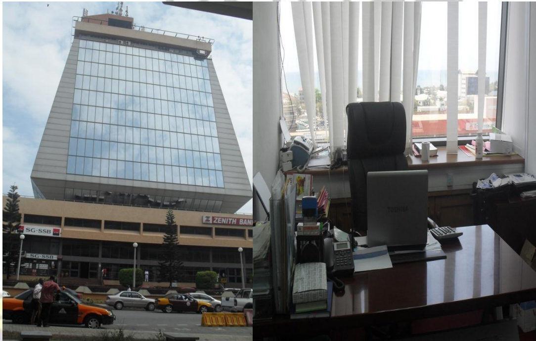
Fig. 3.5: Outdoor and indoor view of selected space in building P.T.
