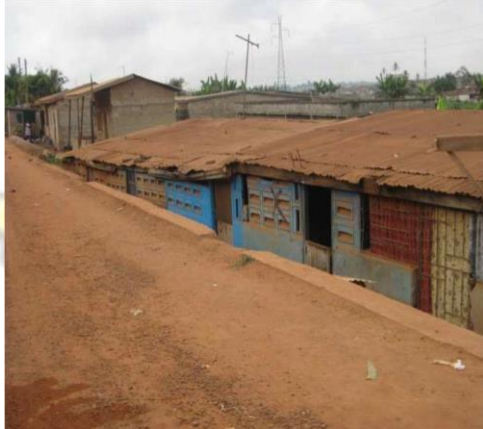
Plate 10: Residential development close to the street marked for demolition
