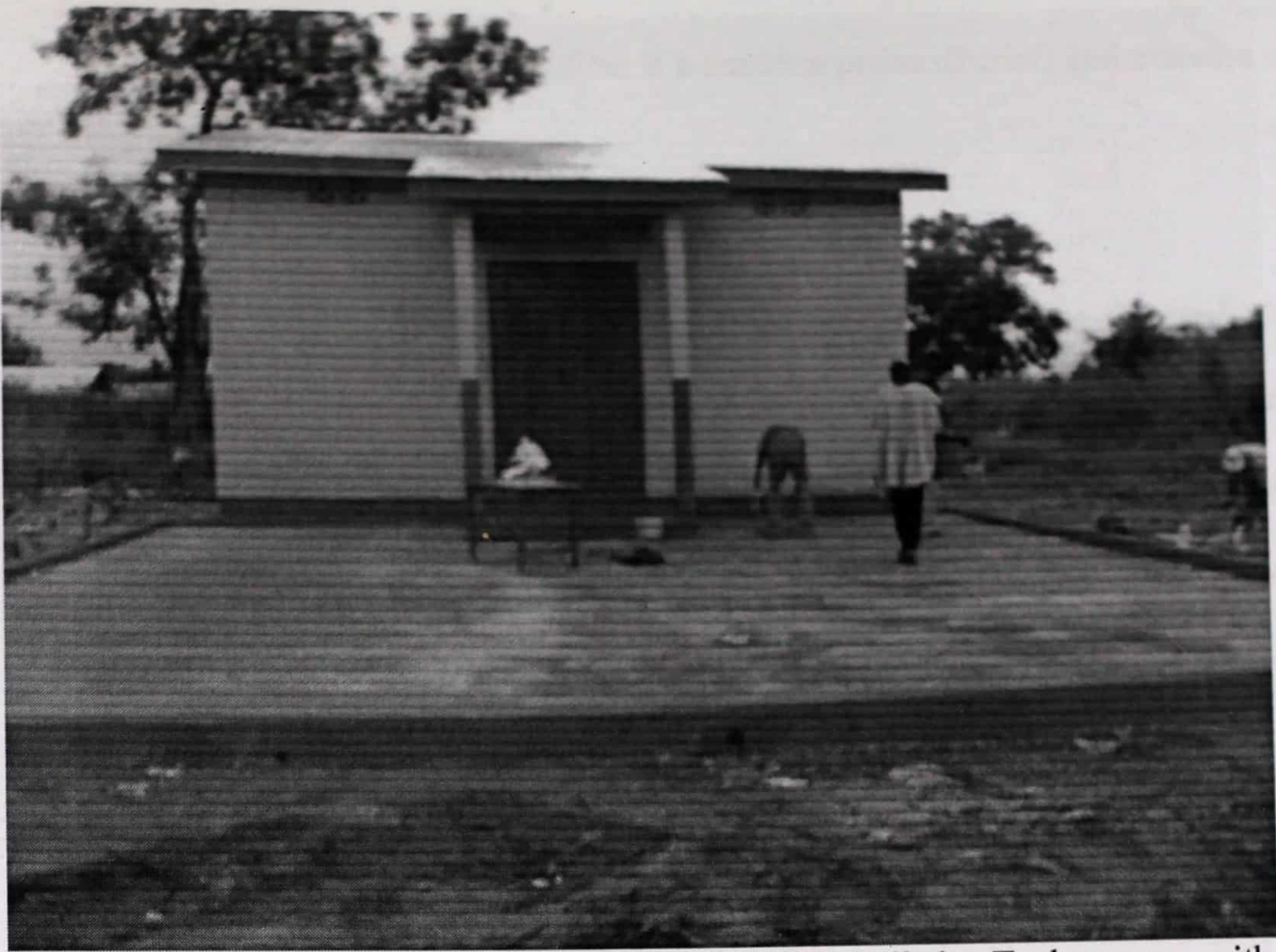
Figure 5.1: A community-managed warehouse built by Technoserve with support from USAID
