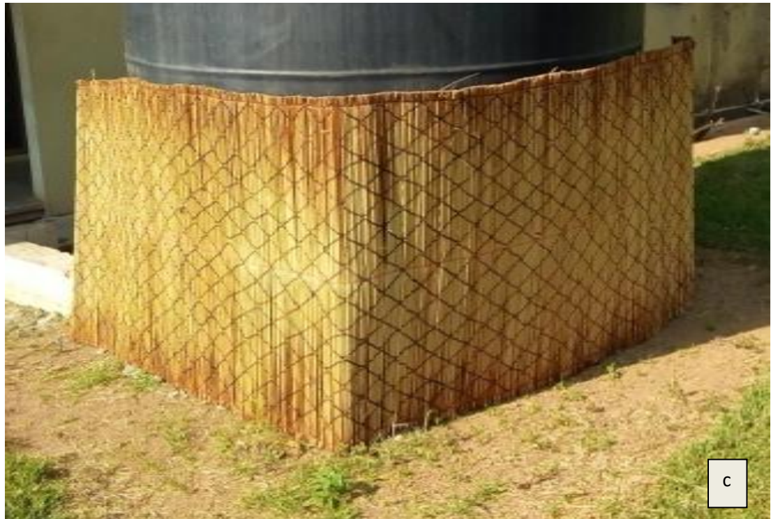
Plate 72 b & c. Final work (Multipurpose wall cover)
