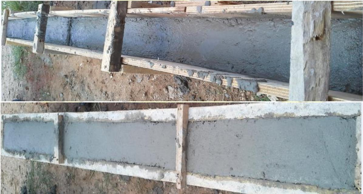
*Fig. 3.8 Samples of cast beams*
