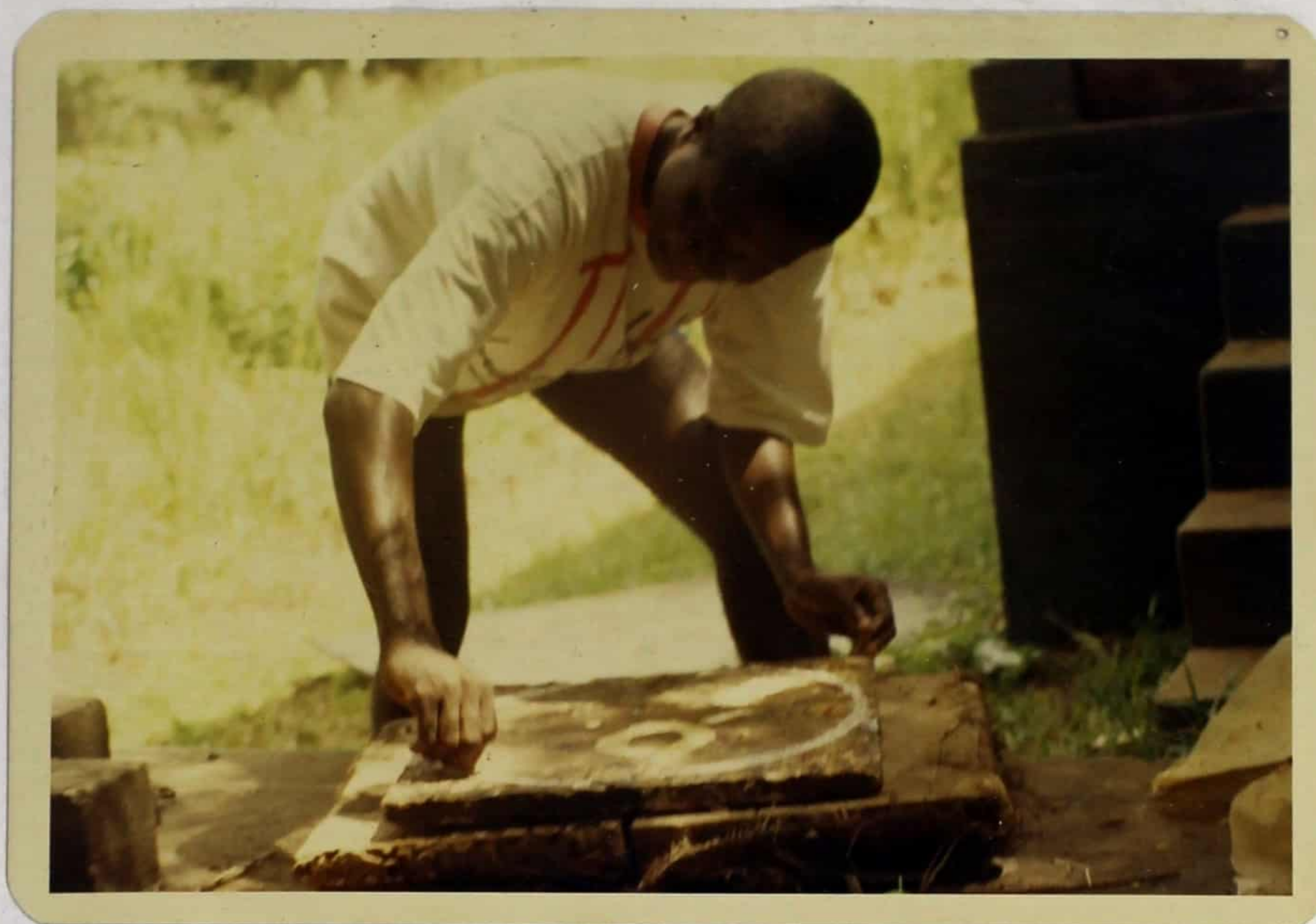
Plate 1. Marking diameter of kiln on the base
