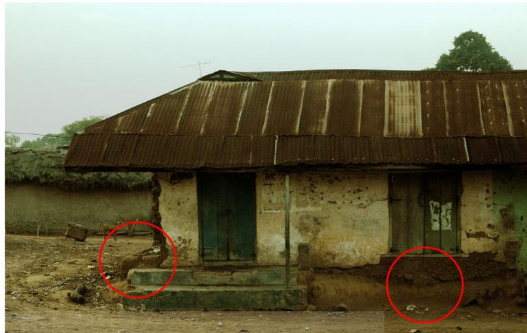
Picture 1 - Materials combination problems. The image shows how the inadequate foundations and erosion have dilapidated the building, in spite of this was built with cement and corrugated metallic sheets.
