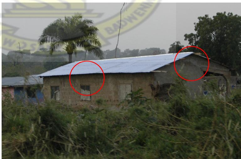
Picture 3 - Roof Design - The use of short eaves do not protect the walls from rain. In particular walls made with some some technique based on raw earth should be protected againt rain and moisture.
