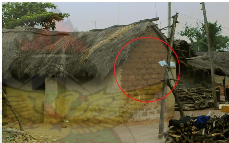
Picture 2 - Materials combination problems. The image shows the union problems of inadequate mixture of cement with adobe blocks. As a result the raw earth wall is rapidly exposed to rain again.
