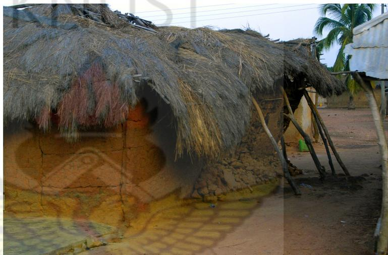
Picture 4 - Degradation of buildings. the surrounding of building lacks from proper drainages and walls are not protected from erosion.
