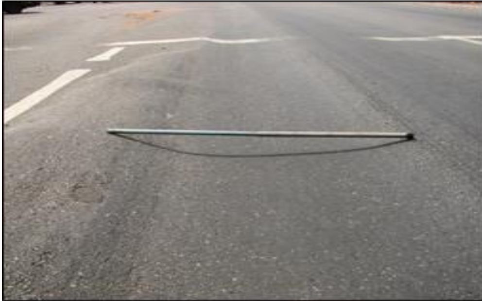
Figure 3-3. Existing 2-lane road showing ruts
