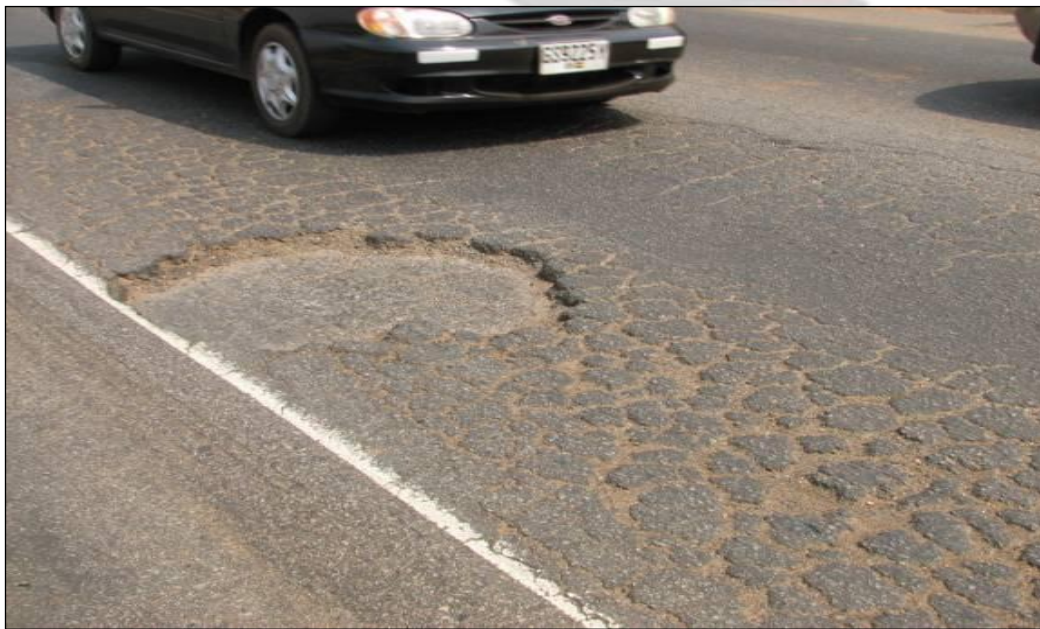
Figure 3-4. Existing 2-lane road showing severe cracks
