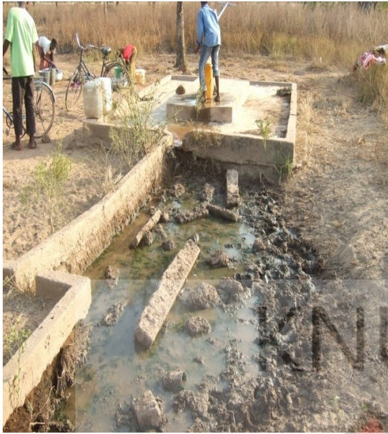
Fig. III: Broken trough with growing algae
