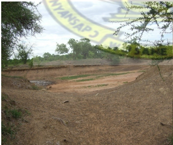
Fig. XXIX: Failure due to overtopping at Bagurugu
