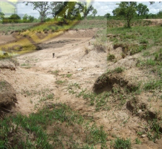
Fig. XXX: Failure due to poor compaction at Pishigu
