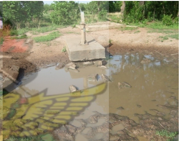
Fig. X: Collapsed trough with mud and water
