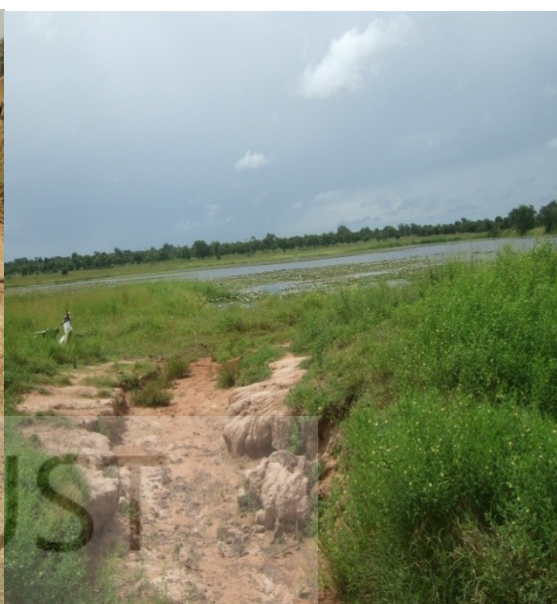
Fig. XXII: Erosion at dugout
