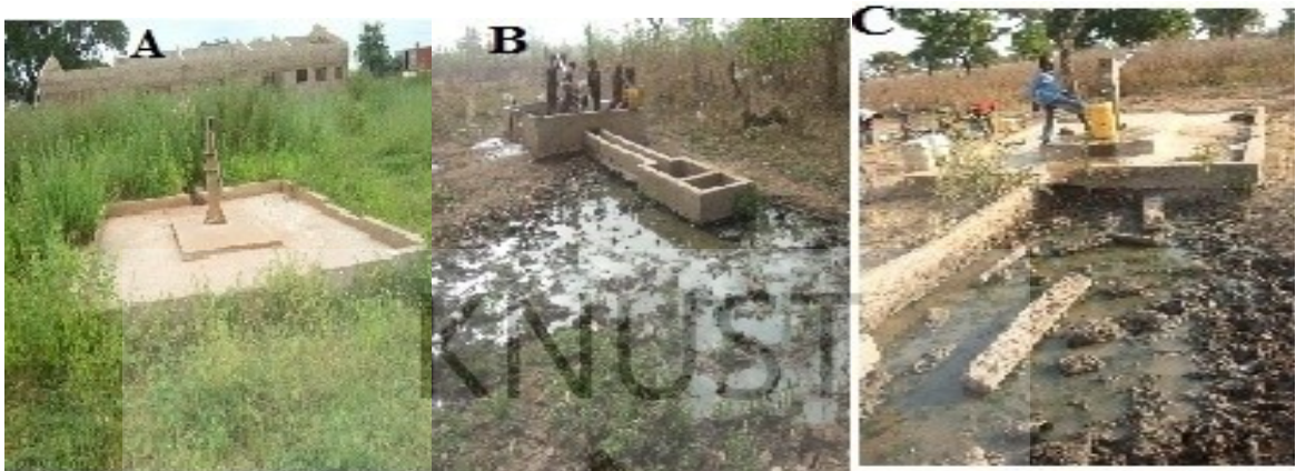
Figure 4.14: Borehole with sanitation threats: scene at (A) Savelugu, (B) Zinindo and (C) Pishigu in Savelugu-Nantong, Gushiegu and Karaga districts respectively
