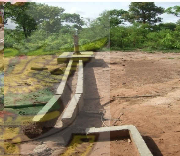
Fig. VI: Broken trough and erosion at BH site
