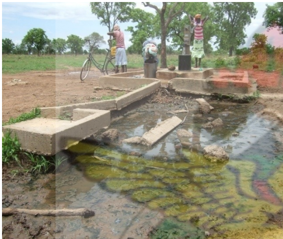
Fig. IX: Broken trough with stagnant water
