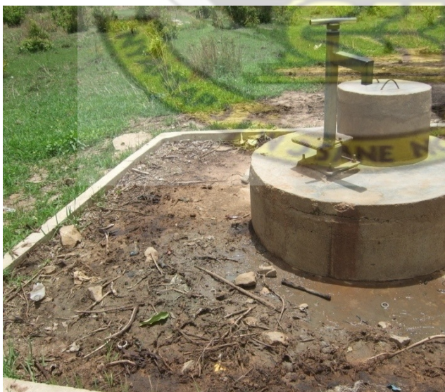
Fig. XI: Dirt and sediments gathered at HDW site
