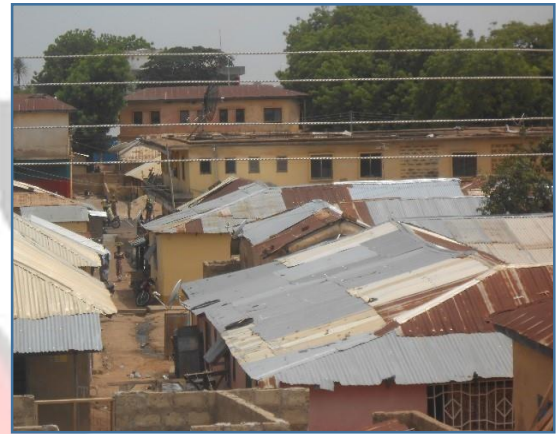
Figure 4.10: Poor access in a residential area
