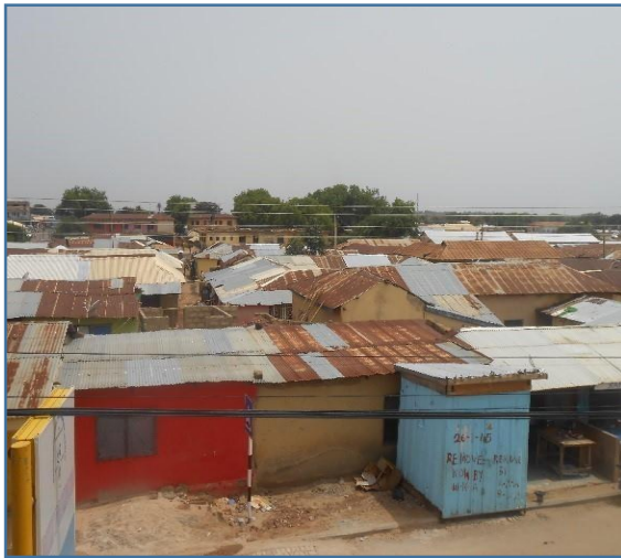
Figure 4.14: Aerial View of Limanyiri
