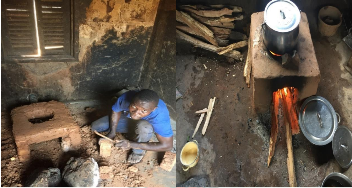
Plate 3.5: Construction and operational phase of improved traditional stove
