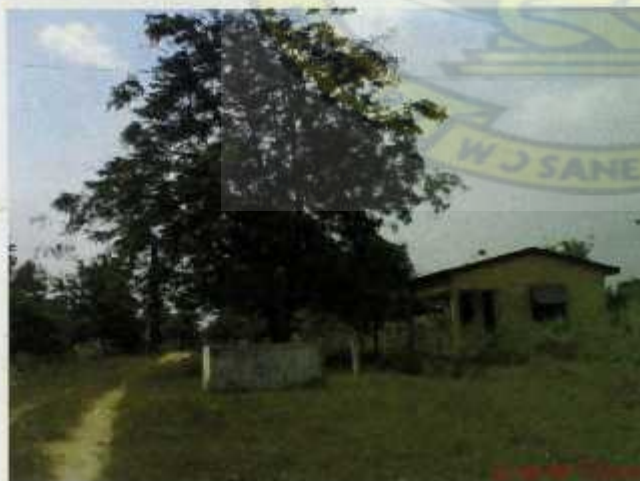
Fig 1.1. Single storey structures scattered across the site
