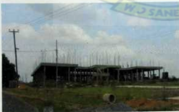
Fig21. C.C.C uncompleted school building
