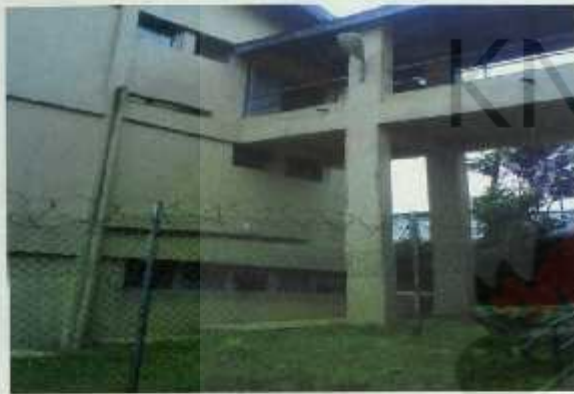
Fig2. Post and beam skeletal frame
