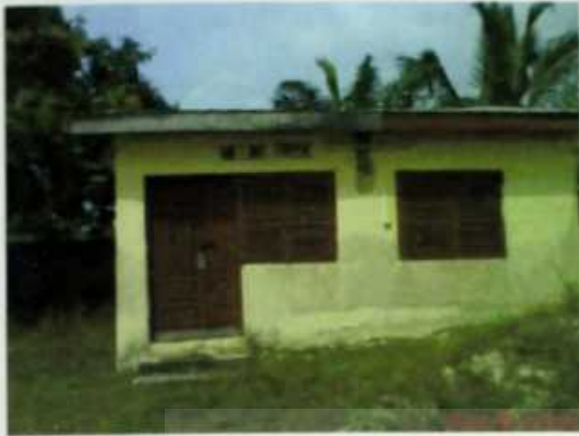
Fig12. Single storey structure with its timber doors and windows
