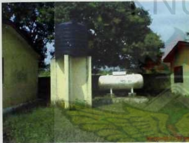
Fig15. Water storage and LPG tank
