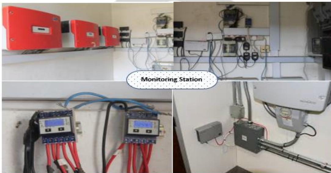
Figure 3-2: Monitoring Station for Outdoor Test Set-up at College of Engineering KNUST, Kumasi, Ghana
