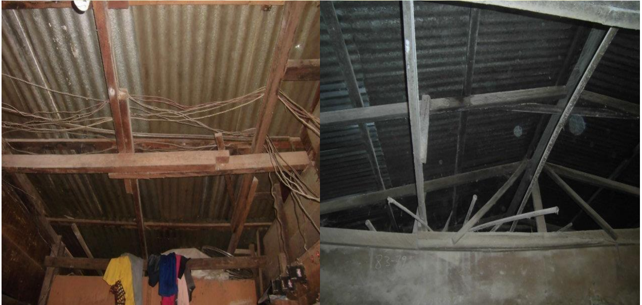
Plate 5: Galvanized aluminium sheet used in roofing without ceiling
