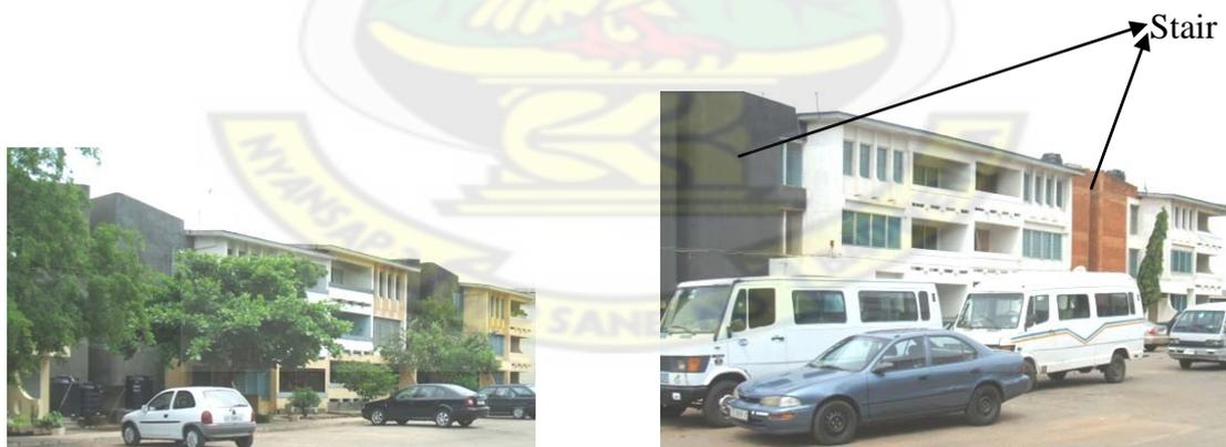
Figure 2.27 The alternative use of brick and Tyrolean finish at stair areas
