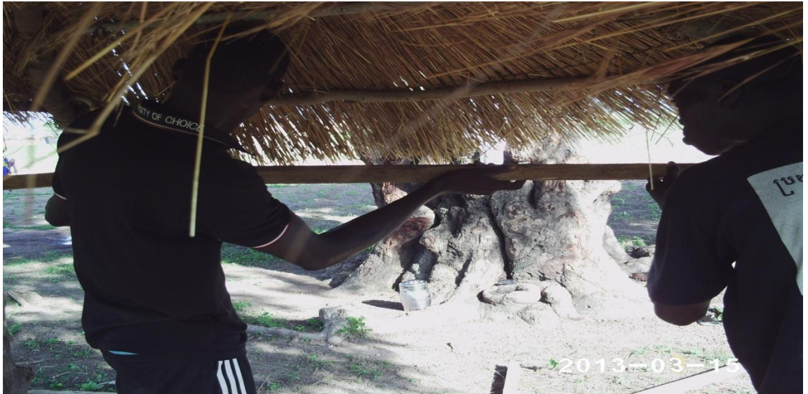
Plate 3: Constructing the structure
