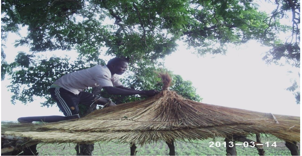
Plate 1: Roofing the evaporative cooler
