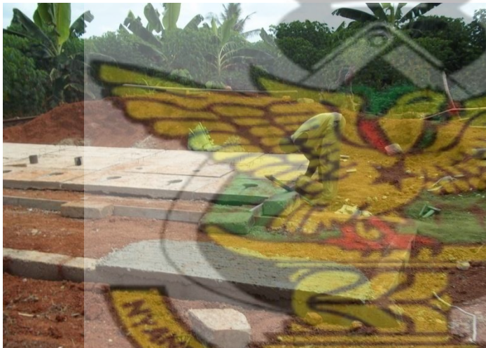
Figure 4.6: Picture of an Ongoing Construction of KVIP Toilet at Fufuo D/A JHS
