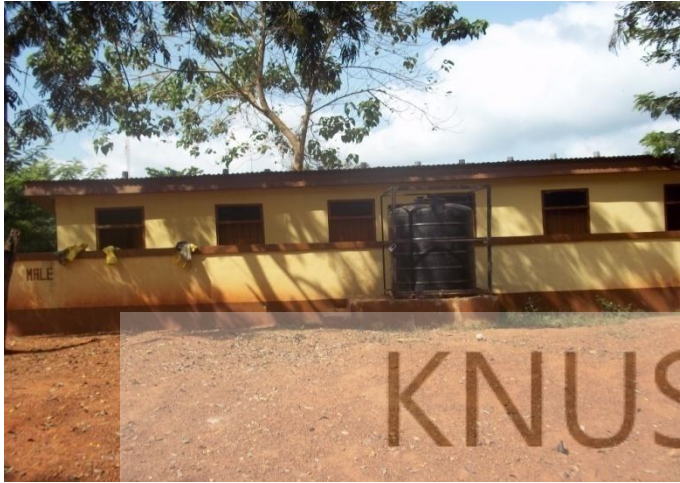
Figure 4.5: A Completed Six Seater KVIP Toilet at Fufuo Methodist Primary
