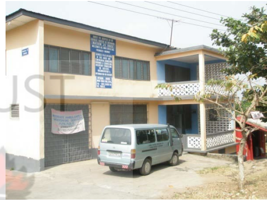
Figure 4.2: The general overview of Matthew 25 House.
