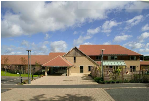
Figure 2.4: The general overview of children's hospice. (Source: children's hospice 2004)
