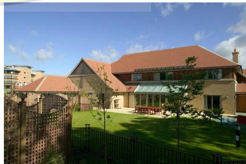
Figure 2.5: The general overview of children's hospice. (Source: children's hospice 2004)
