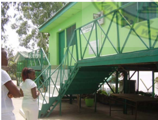
Figure 4.7: Apartments in shades of green
