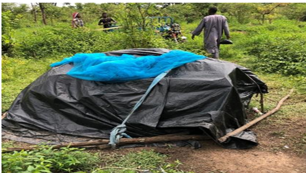
Figure 2.9.4: A wooden housing structure with polythene sheet cover
