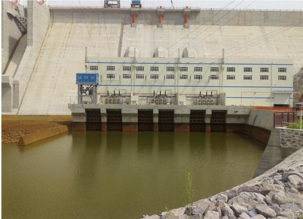
Plate 3.3 Bui Power Generation station showing the three penstocks
