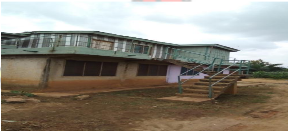
Plate 8.5: Wooden shack constructed on original self-contained flat (Kwadaso) Source: Fieldwork (2017)
