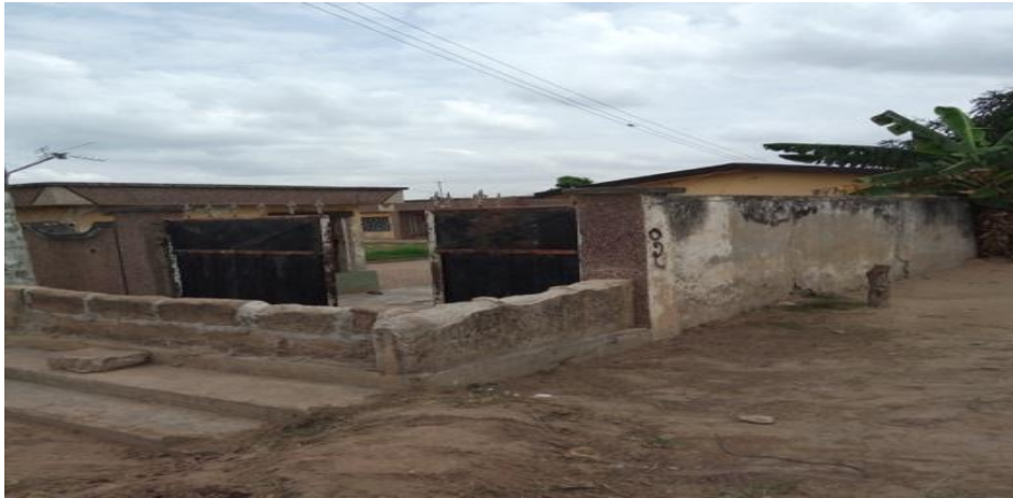
Plate 8.4: Flood defence wall (Atonso S-line) Source: Fieldwork (2017)
