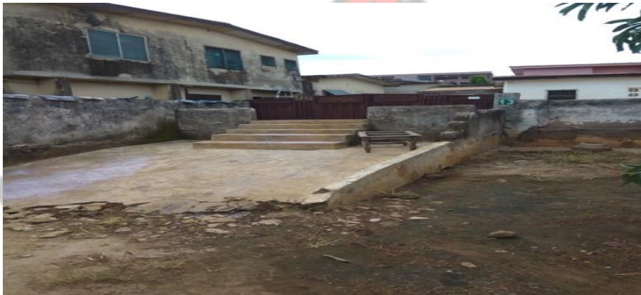
Plate 8.2: Raised concrete entrance with flood defence wall (Kwadaso) Source: Fieldwork (2017)
