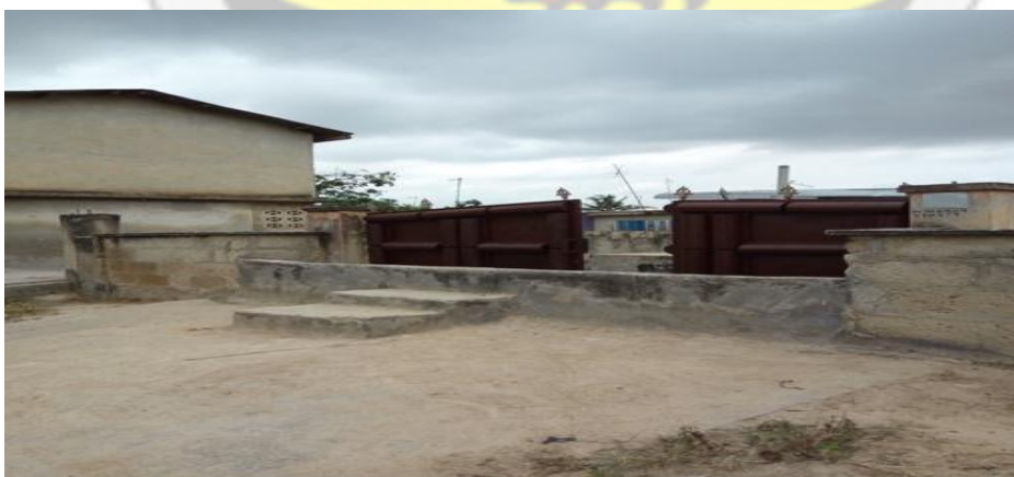
Plate 8.3: Flood defence wall (Breman) Source: Fieldwork (2017)
