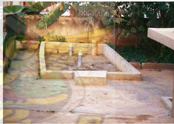
A typical household septic tank with vent pipes showing
