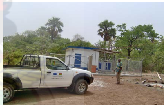
Plate5: standby generator fixed at the pumping station
