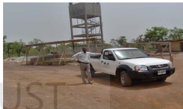
Plate 7: water reservoir near completion
