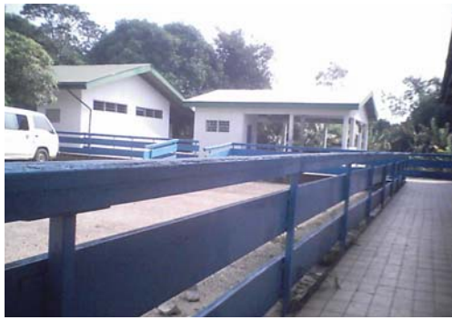
Fig. 4.5 Triple wooden-strip railing
