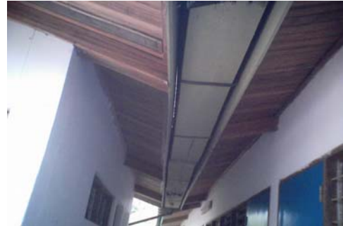
Fig.4.4 Roof gutter for rainwater drainage
