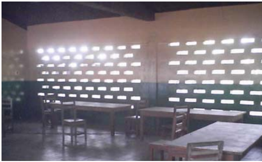
Fig. 4.3 Honey comb walling at the common hall for ventilation and daylighting
