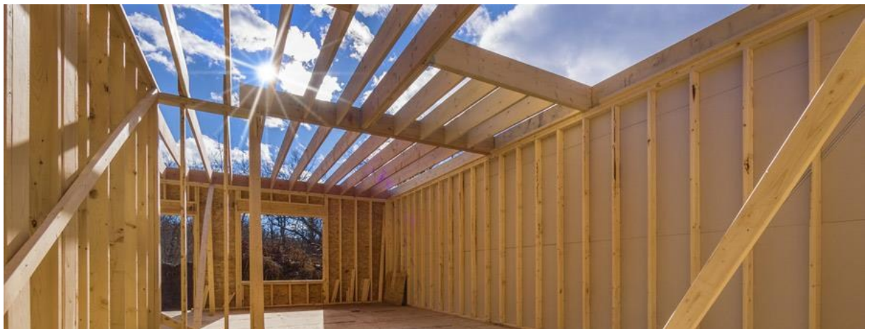
Figure 2.5 Open Panel Timber Frame
