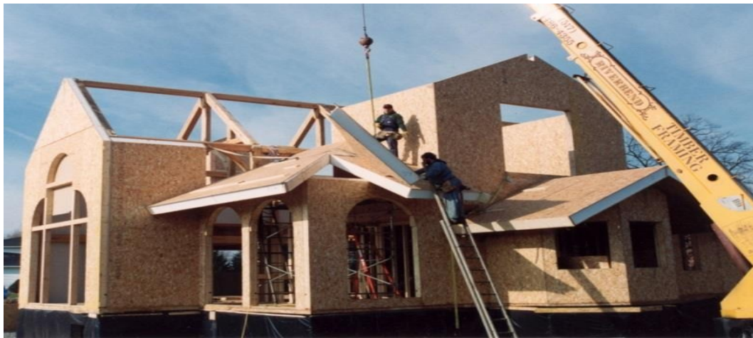
Figure 2.7 Structural insulated panels (SIPS)
