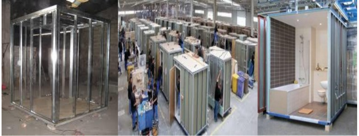
Figure 2.4 Stages in the construction of bathroom pods
