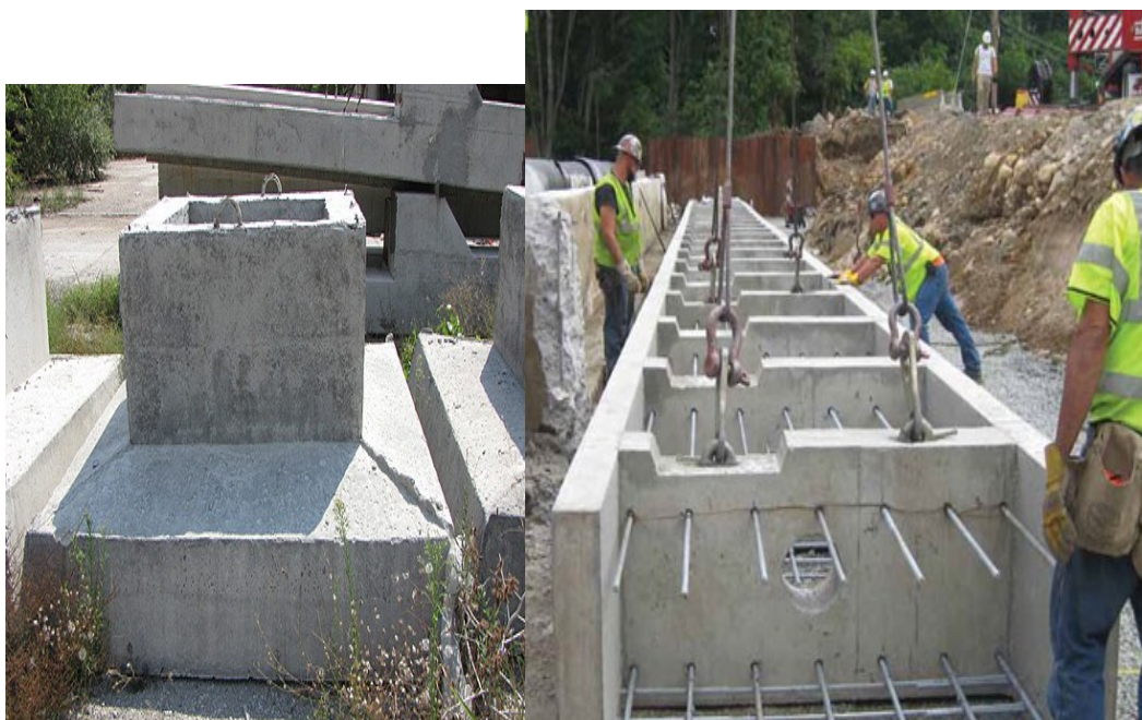
Figure 2.9 Prefabricated Foundation
