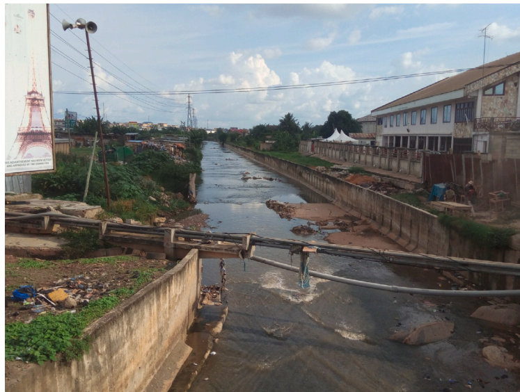
Fig. 6. Flood control channel at Anloga junction in Kumasi, Ghana.
