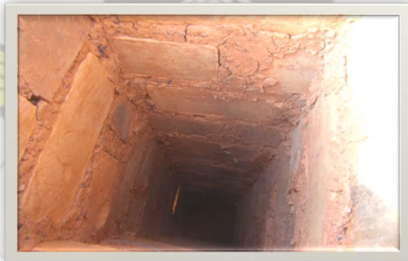
Plate 5.16 The inner part of the chimney after firing
