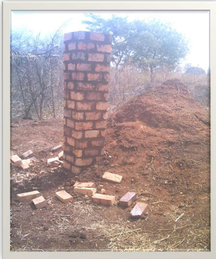
Plate 4.31 Brick chimney of the anthill downdraught kiln
