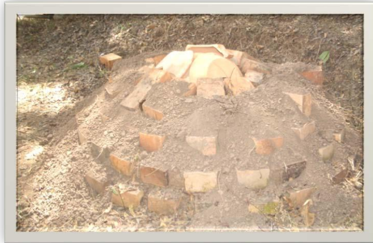
Plate 4.43 Loose soil piled to back up the roof
