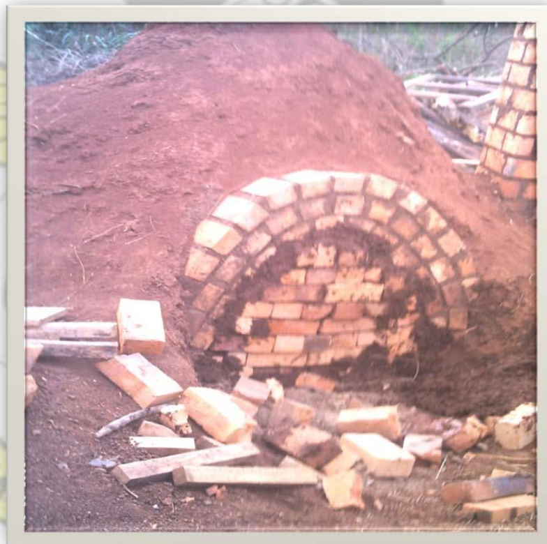
Plate 4.34 Bricked in door of the kiln
