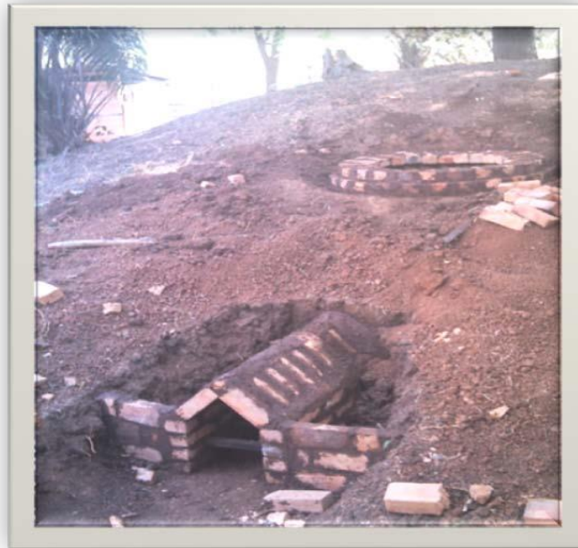
Plate 4.39 Compact mound kiln showing the hearth
