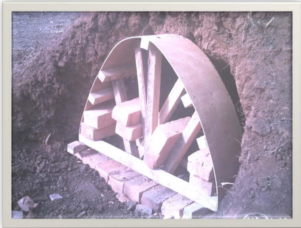
Plate 4.18 Wedge support of the wooden frame
