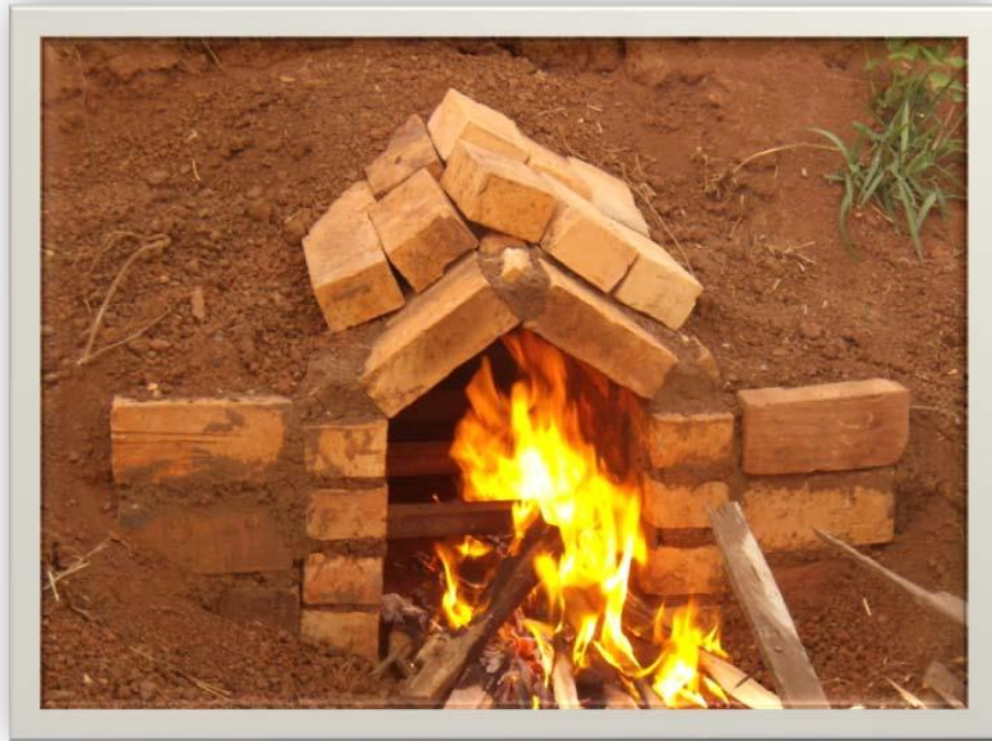
Plate 4.27 Roof of firebox strengthened with bricks.
