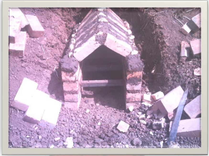
Plate 4.26 Bridge almost complete
