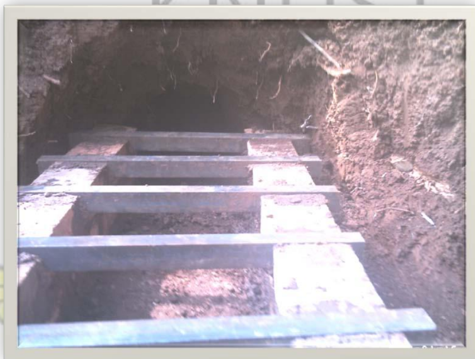
Plate 4.23 Erection of fire bars
