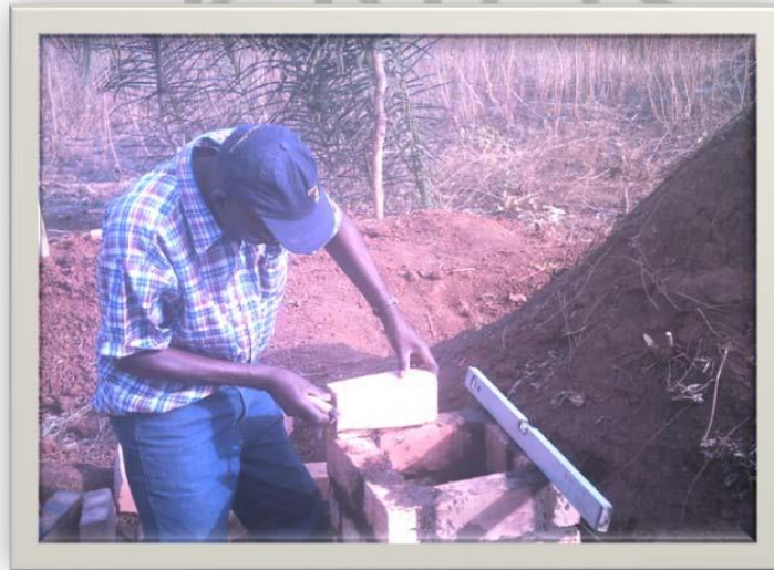
Plate 4.29 Checking the plumb of the chimney
