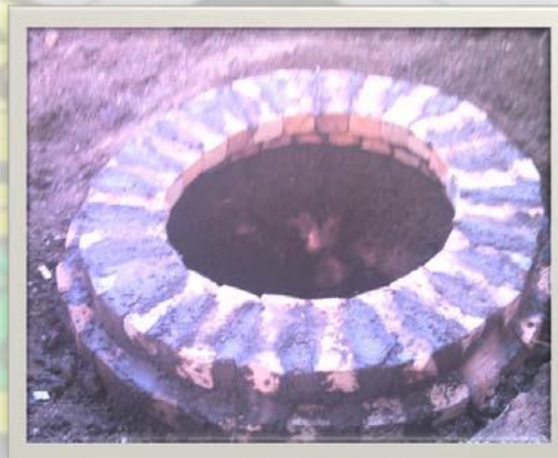
Plate 4.38 Two courses of bricks corbelled to close the mouth
