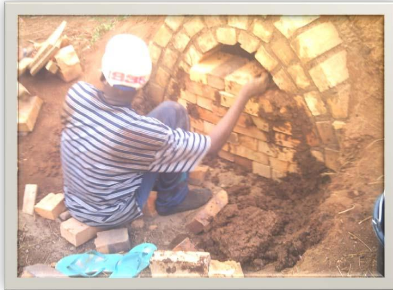
Plate 4.33 Fixing a brick to serve as a spy hole.
