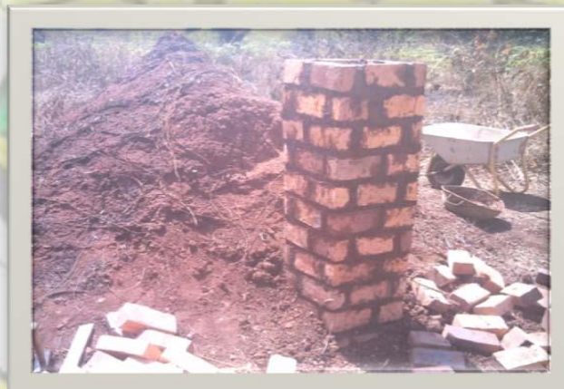
Plate 4.30 Construction of the chimney
