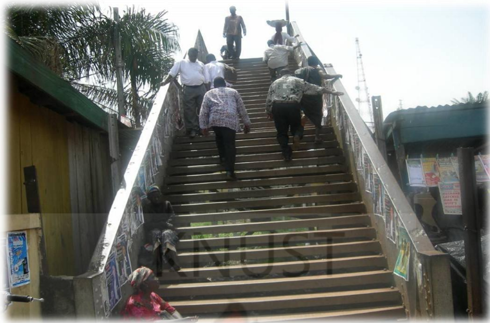
Plate 2.21: The pedestrian walkway over-pass at Railways near Asafo, Kumasi (Source: Appiah-Kubi, 2010)
