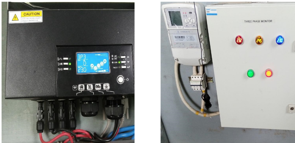
Figure 11. Simulation of generation capacity and output voltage monitoring from AMI (Source: Authors Construct, 2023).
