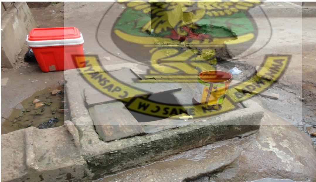
**Plate 4: A shallow hand-dug well covered with a typical wooden cover slab.**
