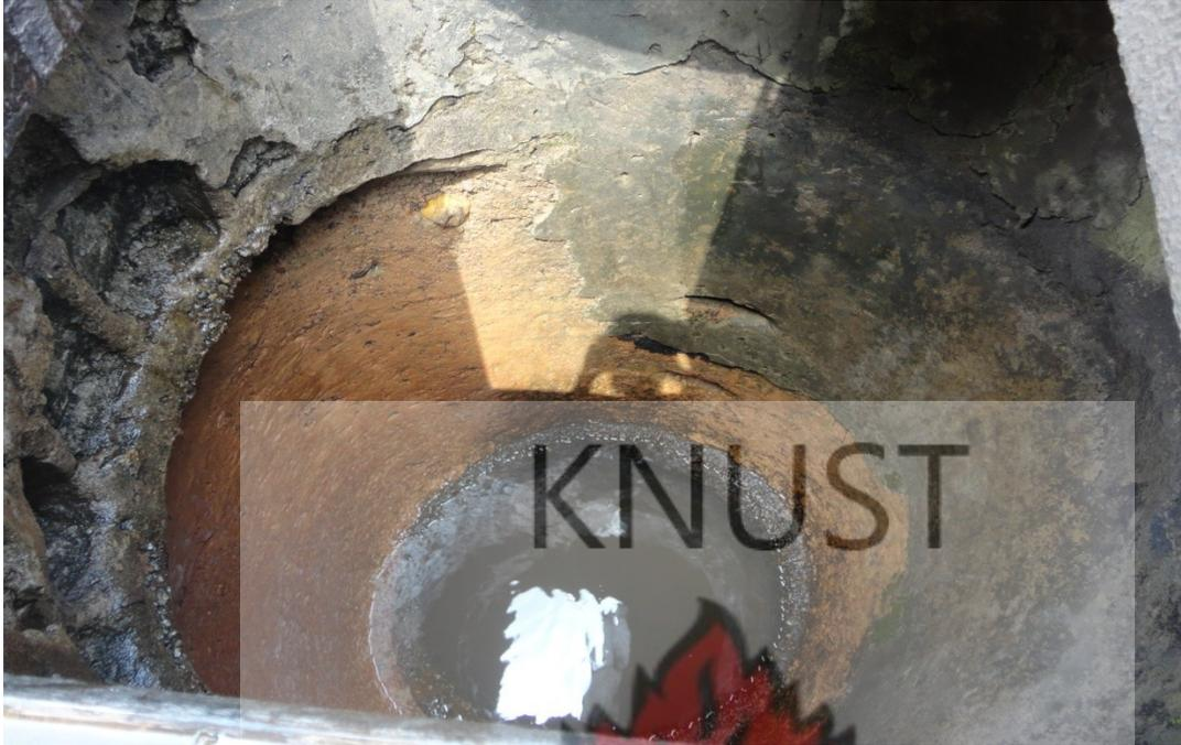
**Plate5: A hand-dug well with fissured concrete lining.**
