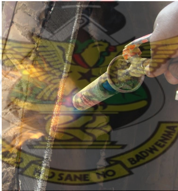
Plate 3.53 Burning off the armature forming the dome
