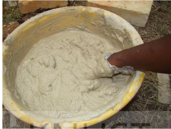
Plate 3.35 Mixing of locally composed kiln mortar
