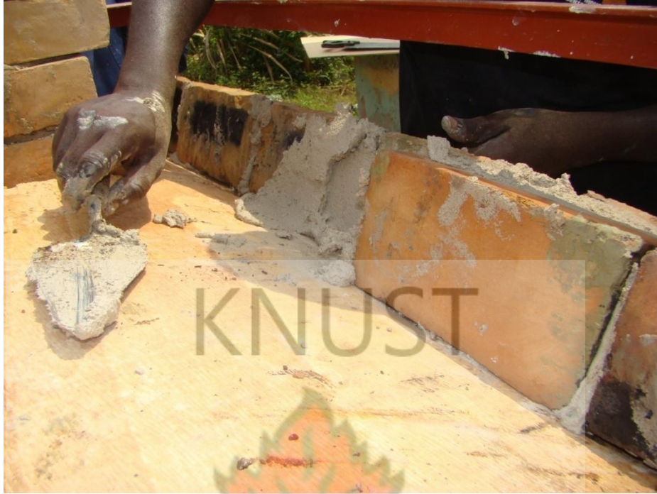
Plate 3.44 Constructing the dome
