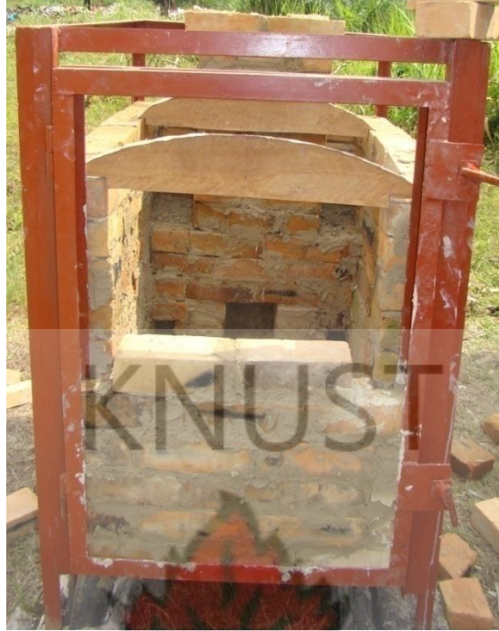
Plate 3.42 Dome framework fixed on top of kiln wall
