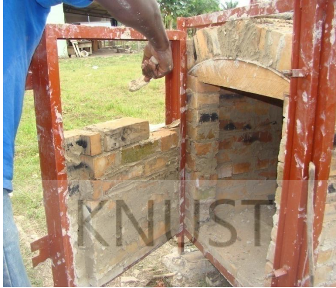
Plate 3.48 Constructing the kiln door
