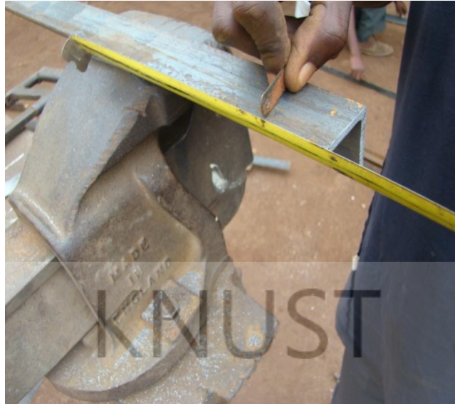
Plate 3.29 Measuring and cutting materials to size
