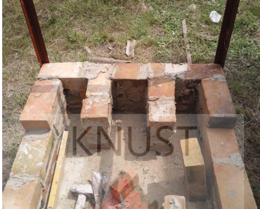
Plate 3.39 Internal walls of the chimney
