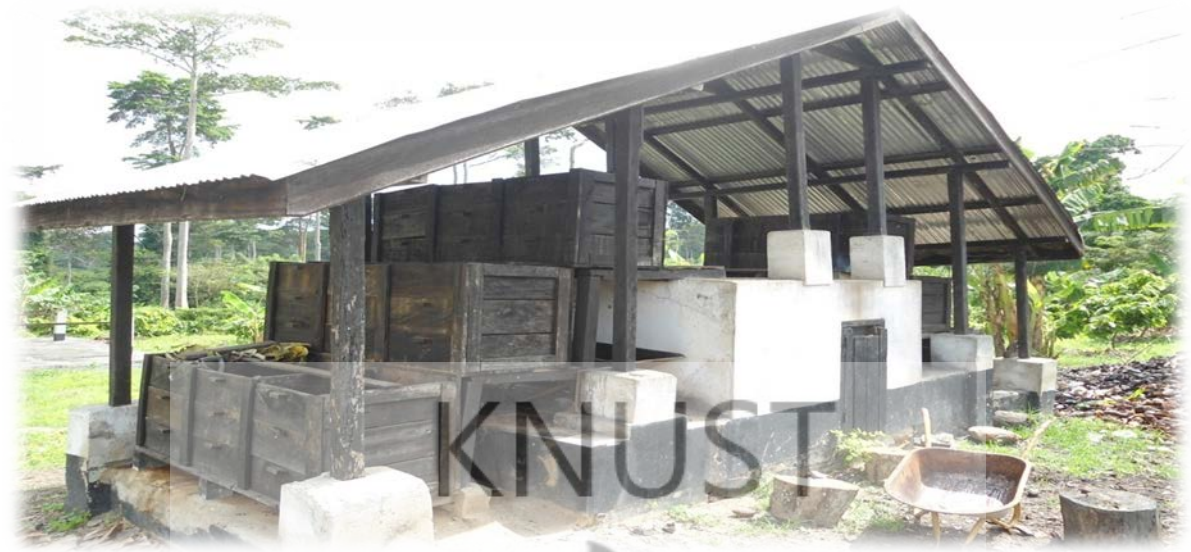
Figure 1: The 3 tier box fermentation system.
