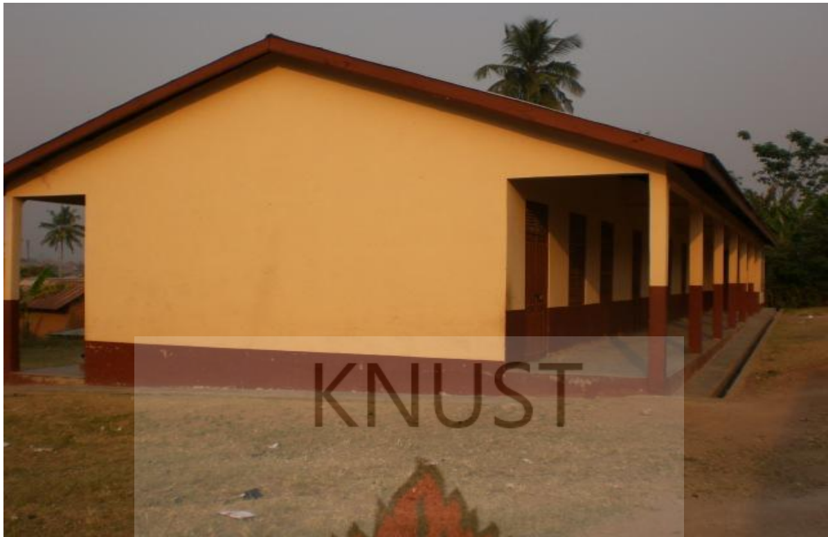
Plate 4.2 - Three-Units Classroom Blocks At Nyaboo
