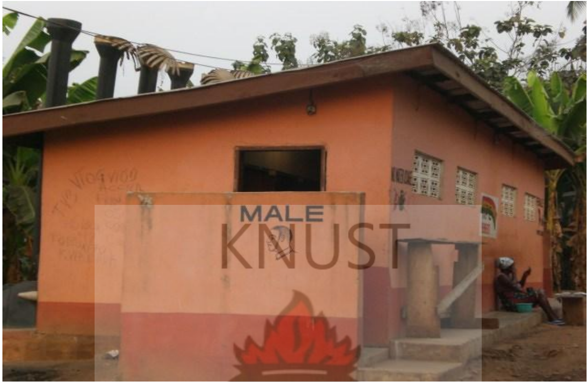
Plate: 4.4 - Six – Seater KVIP at Ananekrom
