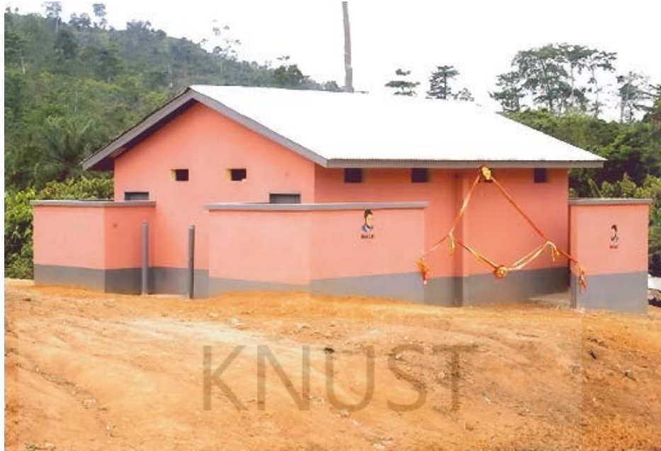
Plate 7 A newly Constructed 12-seater Aqua privy for Etwebo Community in the Chirano Gold Mines Limited Concession Area
