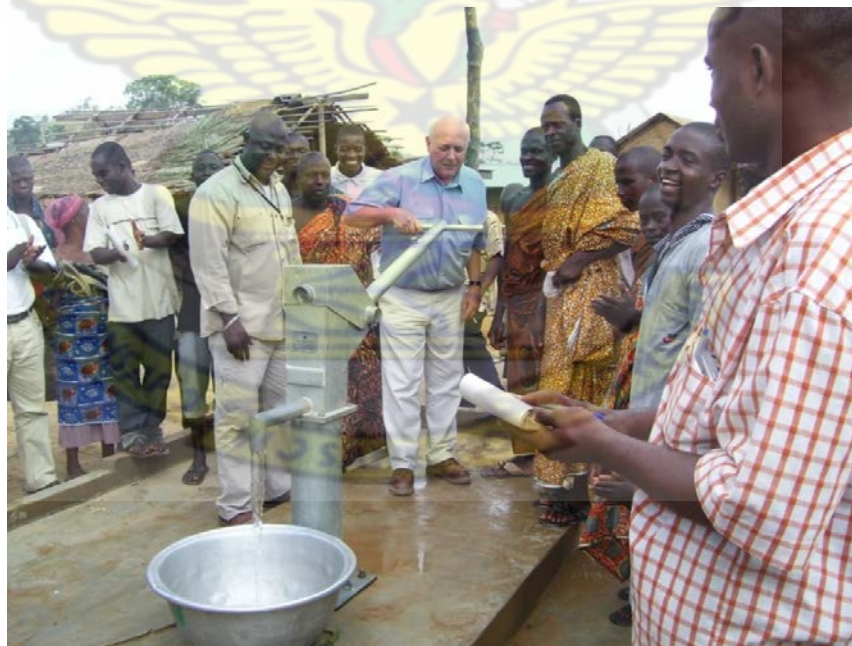
Plate 6: a Borehole Facility for being commissioned by the Akoti Community in the CGML Concession Area
