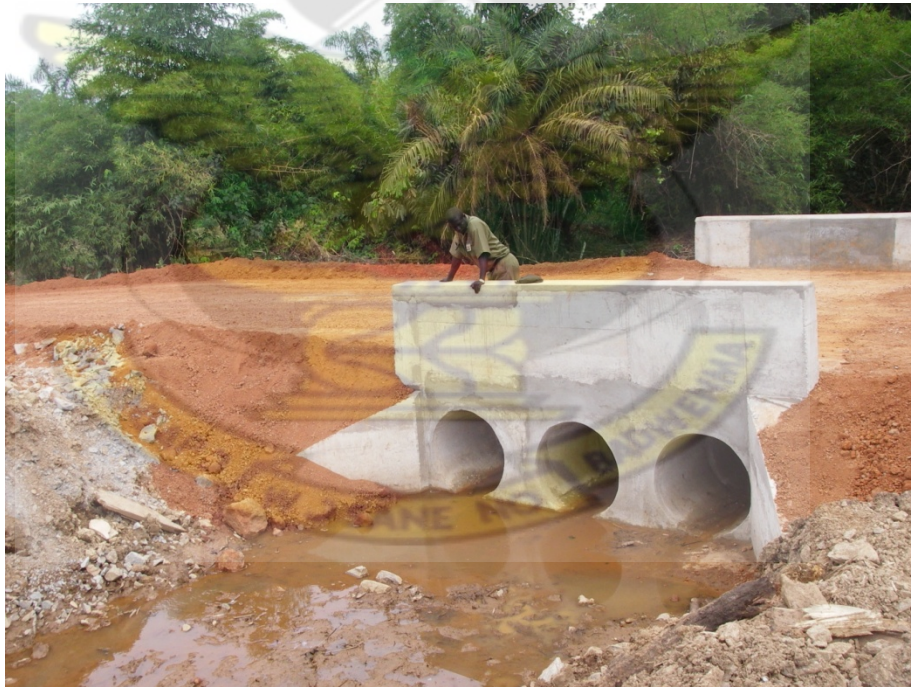
Plate 4b A Newly Constructed Bridge on the Chira River in the CGML Concession Area
