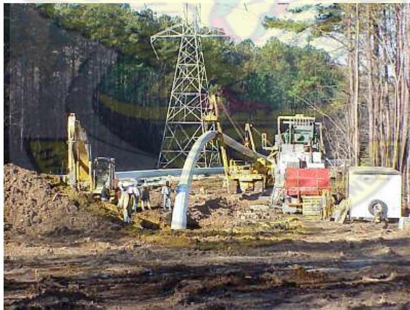
Figure 3.3 Horizontal Directional Drilling (HDD) Operation (Source: Photo courtesy of U.S. Pipeline)
