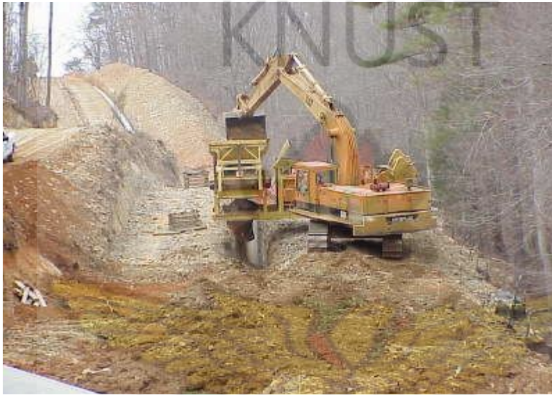
Figure 3.1 Pipeline Trenching Operations (Source: Photo courtesy of U.S. Pipeline)
